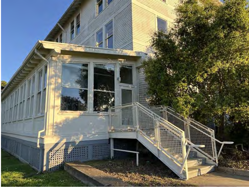
Non Historic Stair at West Elevation, Historic Building 1016
