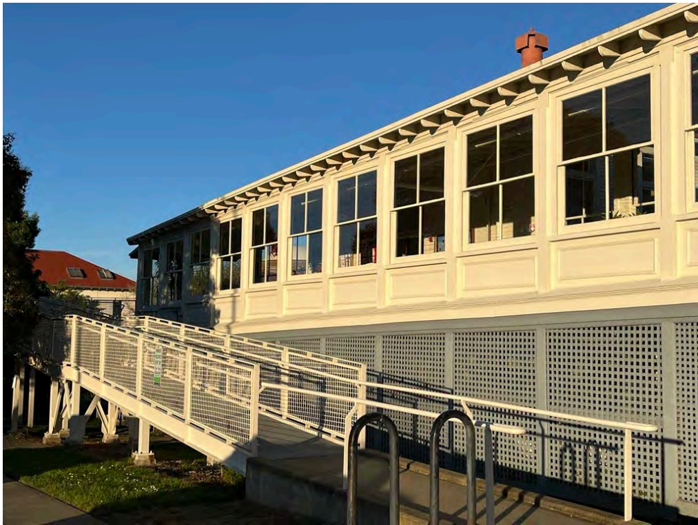
Non Historic Stair at West Elevation Historic Building 1007
