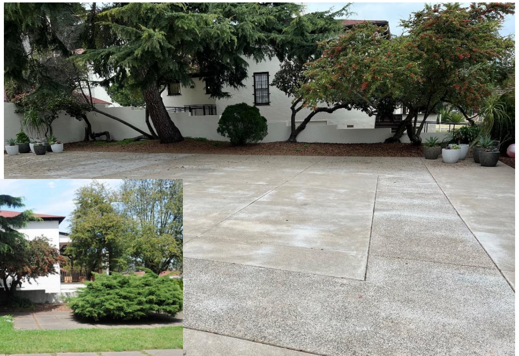
FIGURE 12: BUILDING 45 COURTYARD BEFORE (LEFT) AND AFTER (RIGHT)
