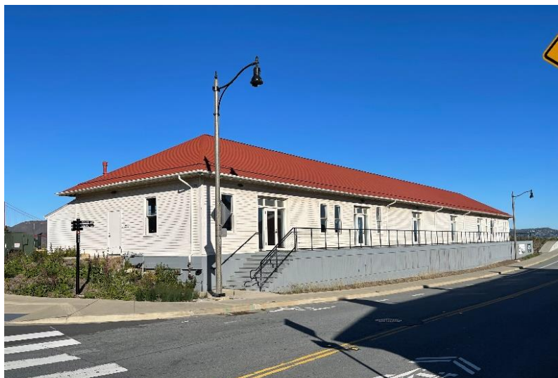
FIGURE 14: LOOKING NORTH AT THE PRIMARY FACADE OF 201 HALLECK STREET
