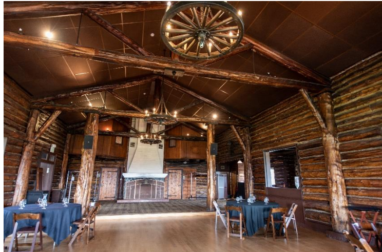
FIGURE 13: LOG CABIN INTERIOR SHOWING ACOUSTIC CEILING TILE TO BE REMOVED
