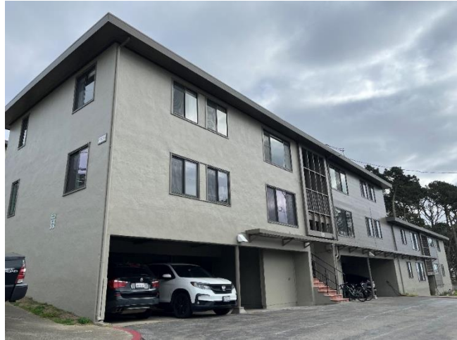
FIGURE 5: BAKER BEACH HOUSING REPLACEMENT WINDOWS IN FOREGROUND, EXISTING WINDOWS IN BACKGROUND
