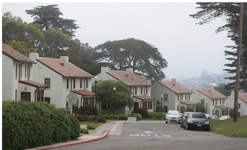
FIGURE 10: STOREY AVE HOUSING WHERE FLOODING FREQUENTLY OCCURS DURING STORMS
