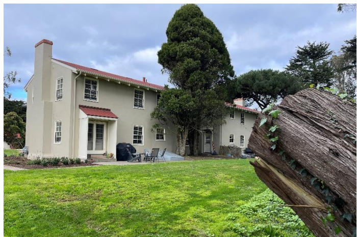
FIGURE 7: 406B E WASHINGTON AFTER REPAIRS
