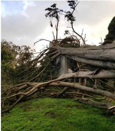
FIGURE 6: 406B E WASHINGTON STORM DAMAGE
