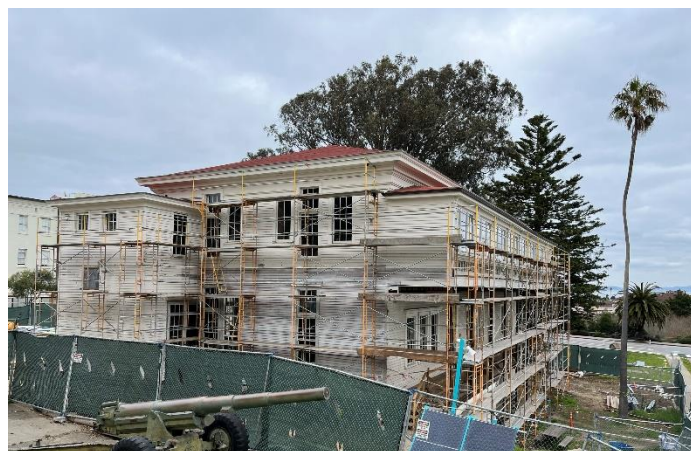
FIGURE 2: BUILDING 2 SURROUNDED BY SCAFFOLDING DURING REHABILITATION
