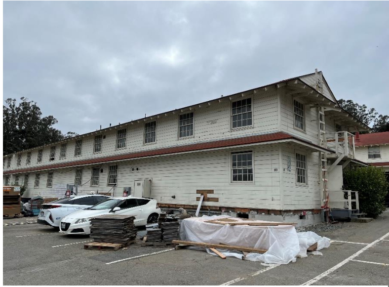
FIGURE 3: LOOKING SOUTHEAST AT BUILDING 40 DURING REHABILITATION
