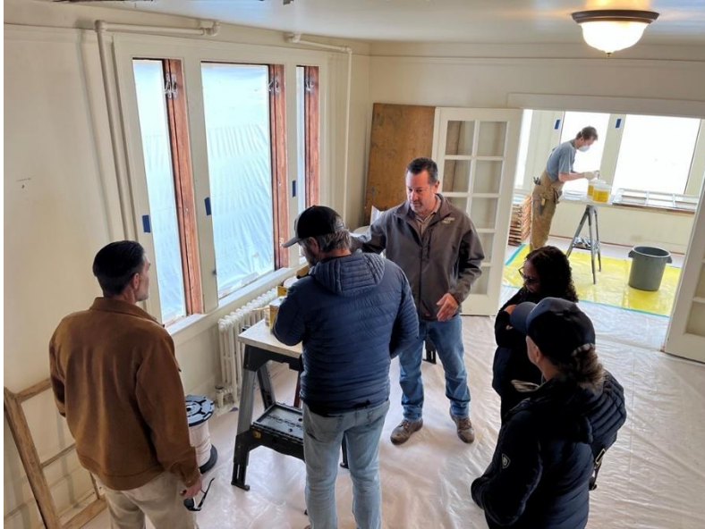
FIGURE 14: PRESIDIO TRUST AND GGNRA STAFF DISCUSS WOOD WINDOW REHABILITATION IN DECEMBER 2025
