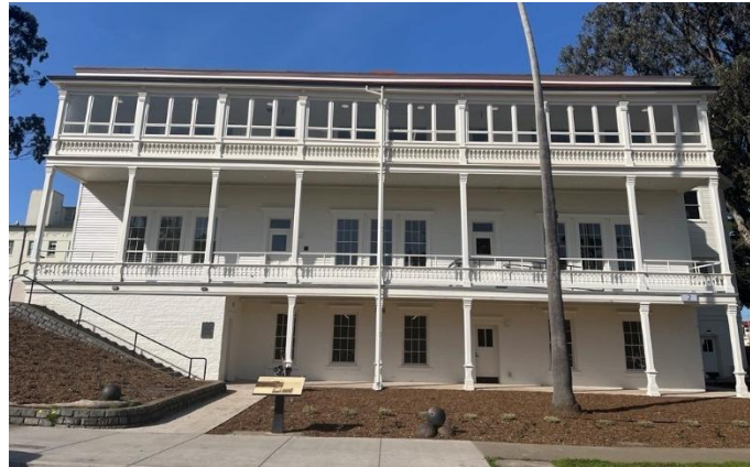
FIGURE 2: REHABILITATED EAST PORCH OF BUILDING 2, OLD POST HOSPITAL
