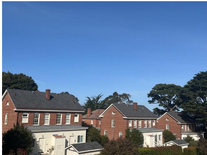
FIGURE 6: EAST REILLY AVENUE RESIDENCES AFTER INSTALLATION OF GREY ASPHALT SHINGLE PILOT
