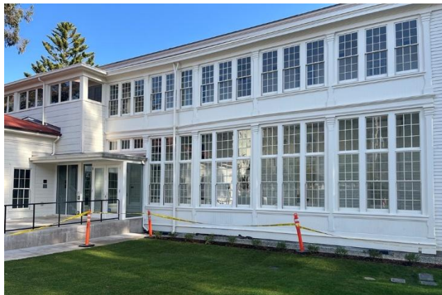
FIGURE 5: REHABILITATED WEST FACADE OF BUILDING 2, OLD POST HOSPITAL
