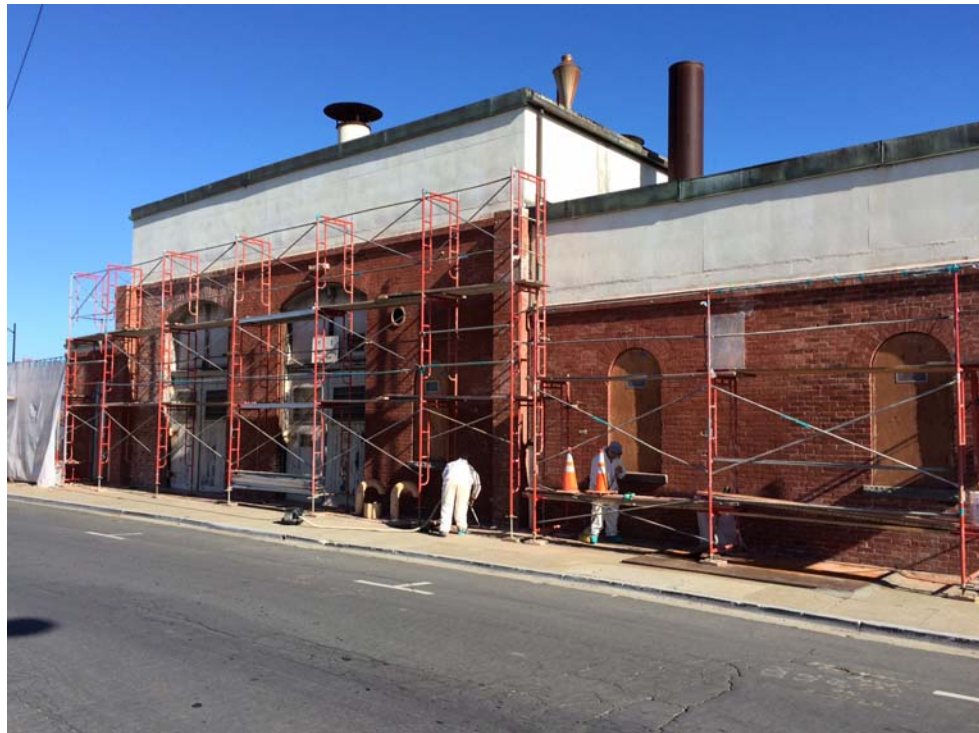
Paint stripping underway at building 1040 as part of the larger preservation maintenance program in the Thornburgh District.
