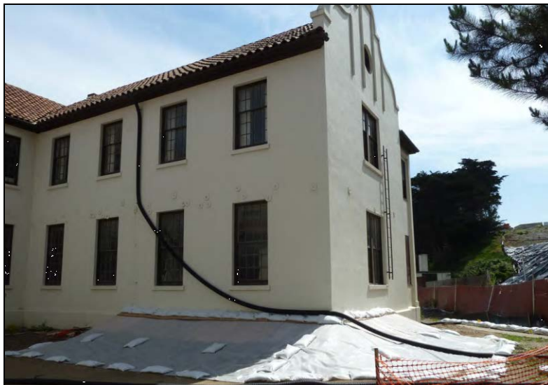
Temporary shoring and protective measures in place. (2014)
