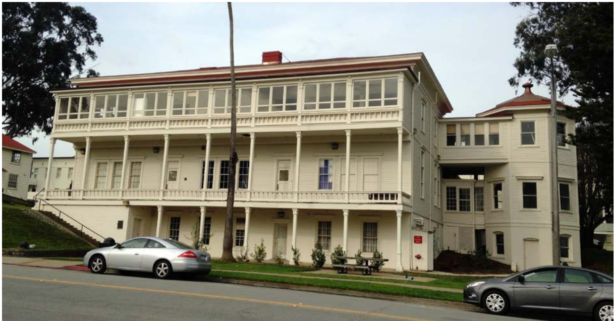
West Elevation of Building 2 (2015)
