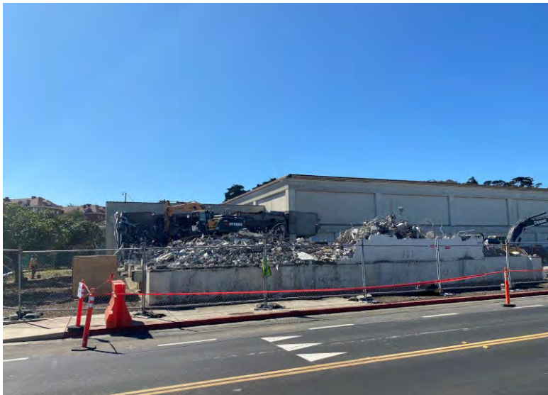
FIGURE 8: BUILDING 653 DURING DEMOLITION
