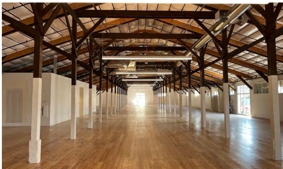
FIGURE 6: INTERIOR OF MASON STREET WAREHOUSE AFTER REHABILITATION.
