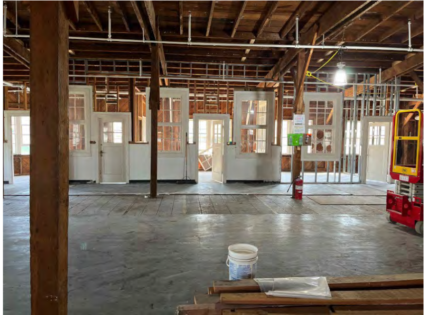
FIGURE 5: INTERIOR OF MASON STREET WAREHOUSES DURING REHABILITATION.
