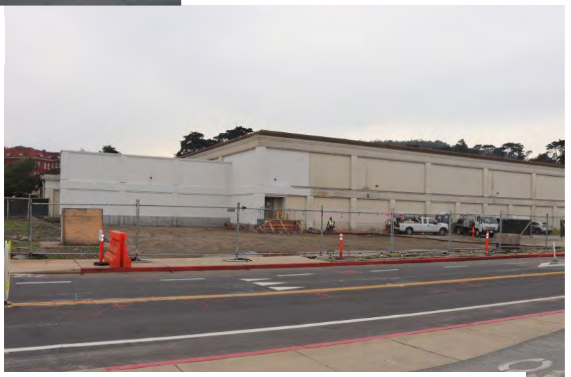
FIGURE 9: BUILDING 610 WITH BUILDING 653 REMOVED.
