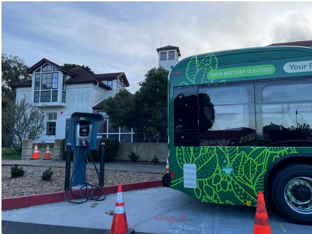
FIGURE 8: ELECTRIC BUS CHARGING STATION
