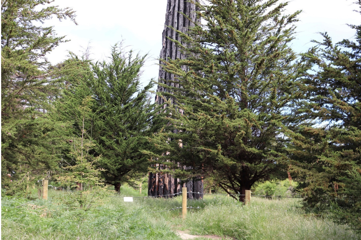
FIGURE 5: “SPIRE” FOLLOWING REPAIRS AND PUBLIC ACCESS RESTRICTIONS
