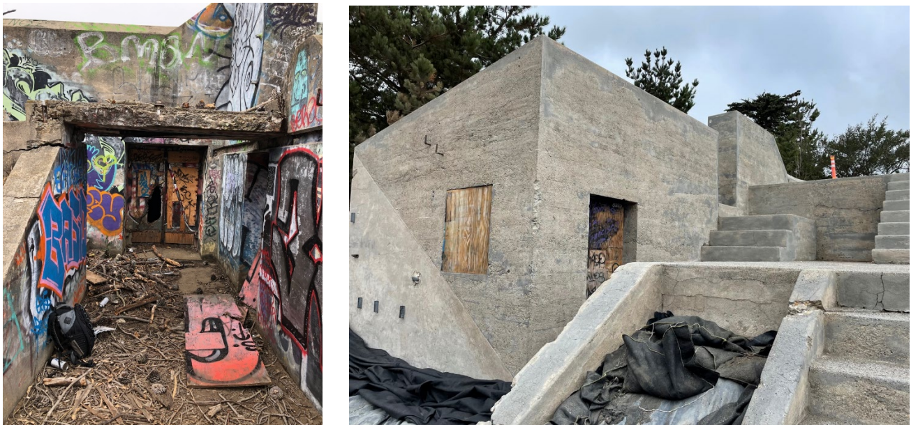
FIGURE 2: BATTERY SHERWOOD BEFORE (LEFT) AND AFTER (RIGHT) CONSERVATION TREATMENTS & GRAFFITI REMOVAL
