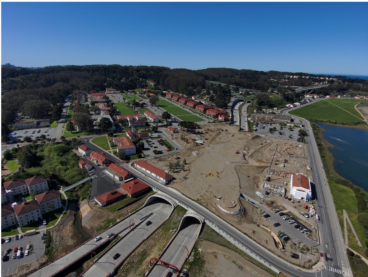
FIGURE 6: TUNNEL TOPS AERIAL, MARCH 2021 (STEPHAN PARK, PRESIDIO TRUST)
