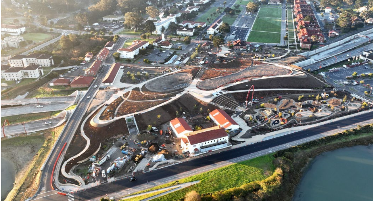
FIGURE 7: TUNNEL TOPS AERIAL PHOTO, DECEMBER 2021
