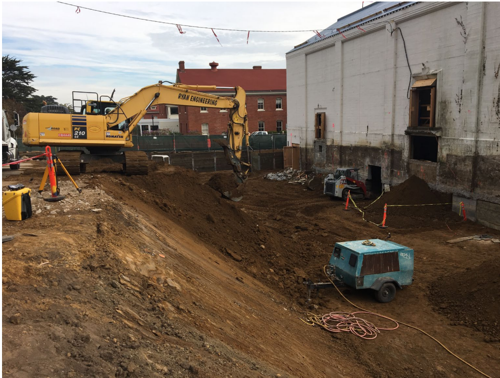
Figure 2 Excavation for the below grade portion of the project (Presidio Trust, January 2018)
