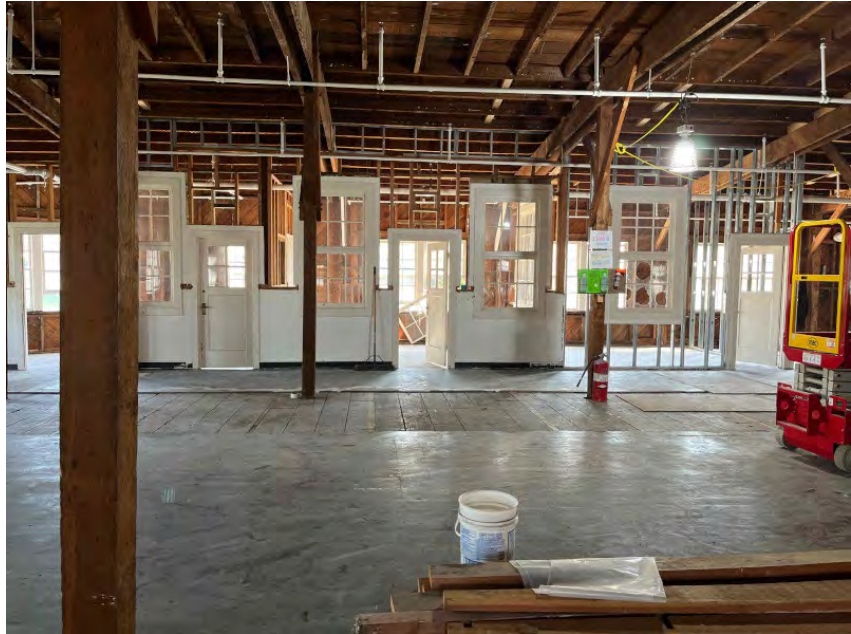
FIGURE 5: INTERIOR OF MASON STREET WAREHOUSES DURING REHABILITATION.
