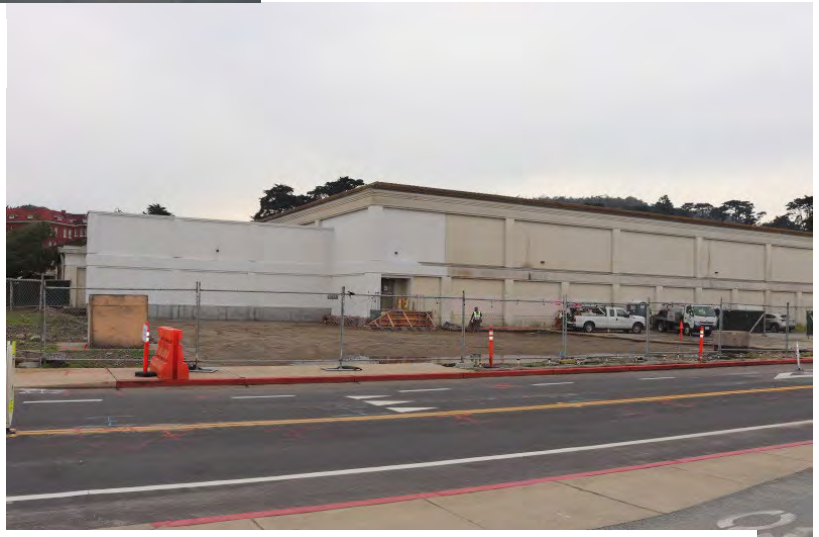
FIGURE 9: BUILDING 610 WITH BUILDING 653 REMOVED.
