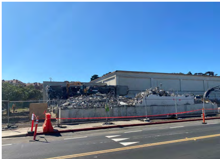
FIGURE 8: BUILDING 653 DURING DEMOLITION
