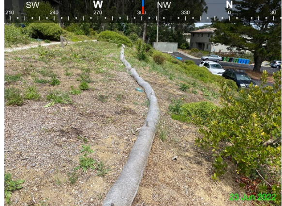
Photo 18: 6/23/2022 – View of vegetated slope, erosion blanket, and former planter box area to the northeast of Building 1257.
