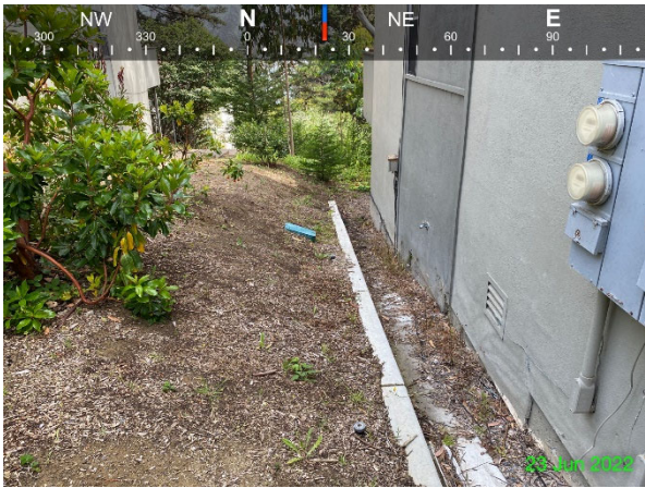
Photo 1: 6/23/2022 – View of intact hardscape and drainage from southwest corner of Building 1279.
