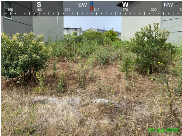
Photo 3: 6/23/2022 – View of vegetated cap between buildings 1278 and 1279. Evidence of burrowing activity is present in the foreground.
