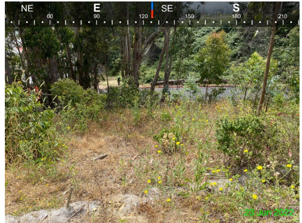
Photo 8: 6/23/2022 – View of the vegetated slope and healthy vegetated cap to the east of Building 1259.
