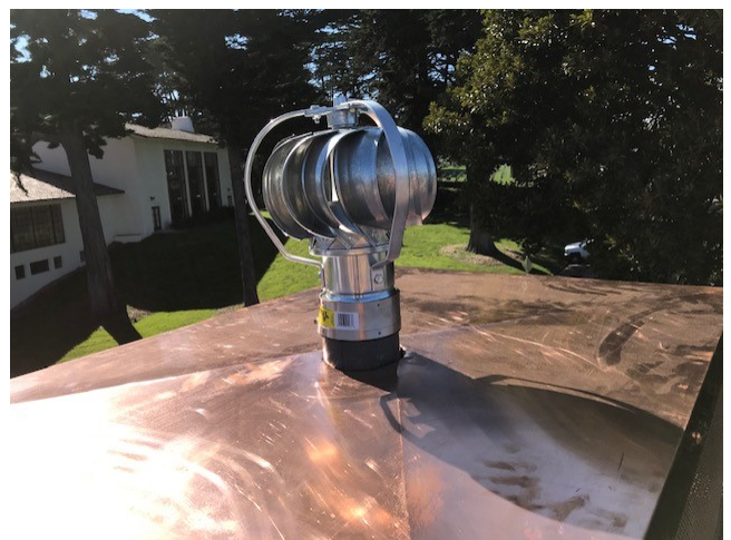
Photo 36: Wind-driven Ventilator
