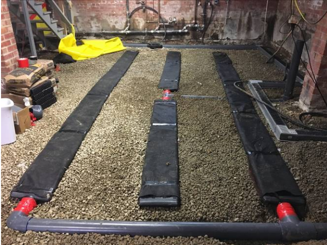
Photo 7: VMS Piping Installation
