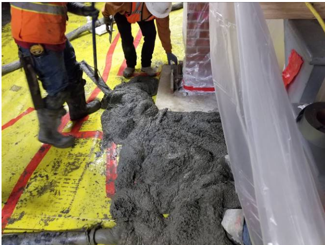
Photo 17: Concrete slab installation.
