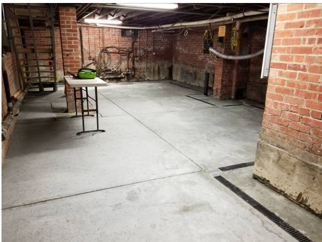
Photo 29: Concrete Slab (cured)
