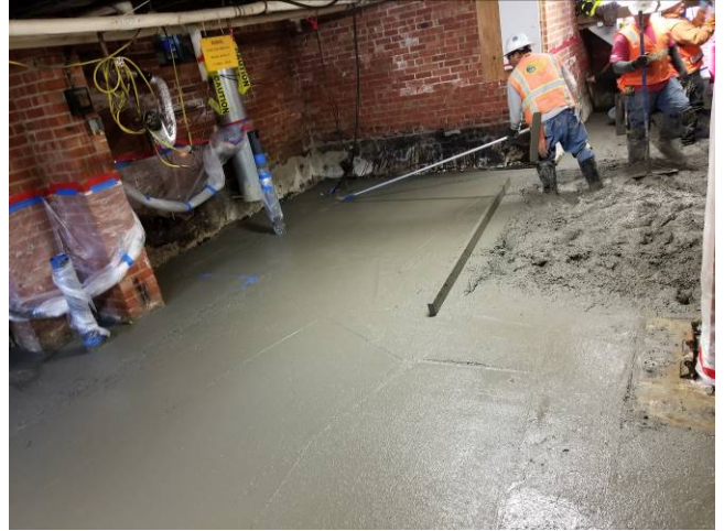
Photo 20: Concrete Slab Installation
