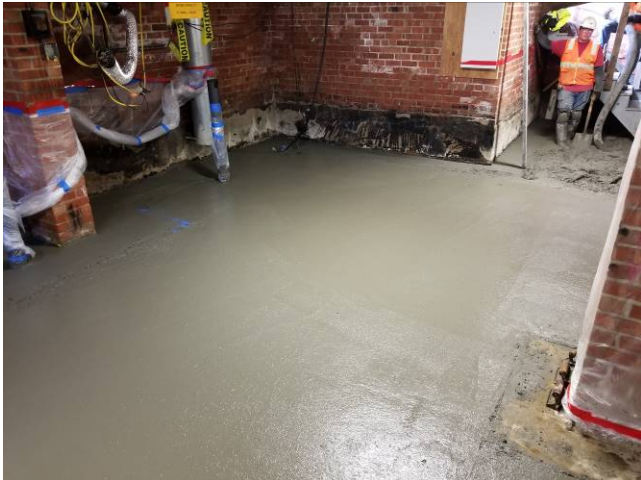
Photo 21: Concrete Slab Installation
