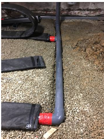
Photo 5: VMS Piping Installation
