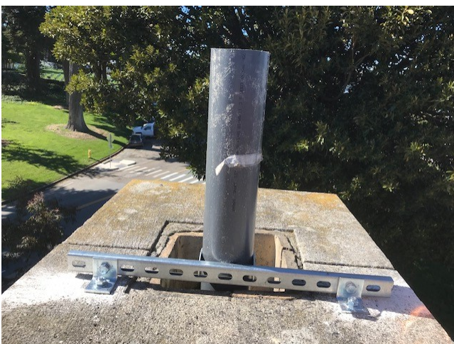
Photo 35: Vent Riser (top of chimney)
