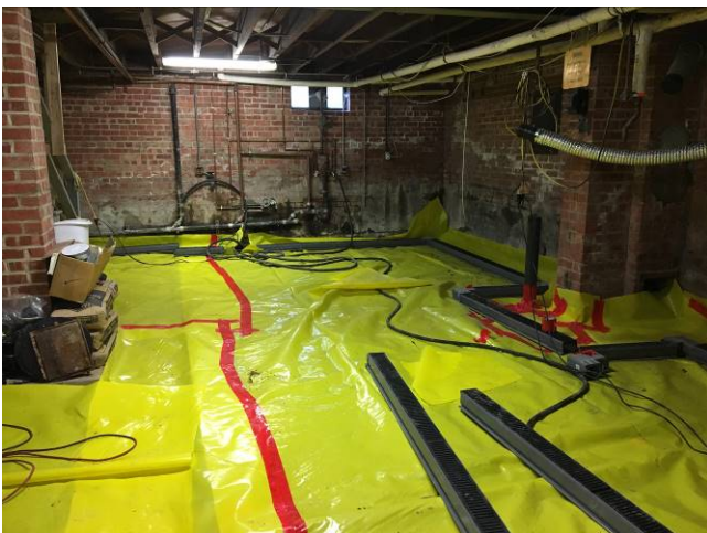
Photo 11: Vapor Barrier Installation
