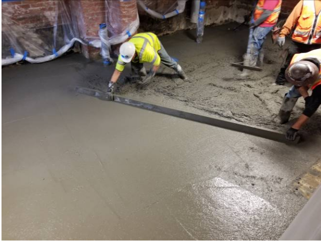
Photo 19: Concrete Slab Installation
