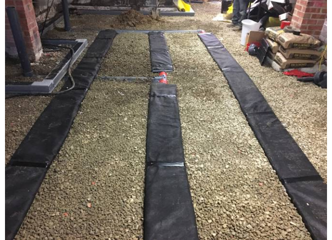
Photo 8: VMS Piping Installation
