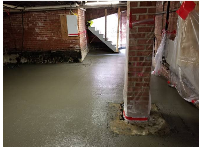
Photo 22: Concrete Slab Installation
