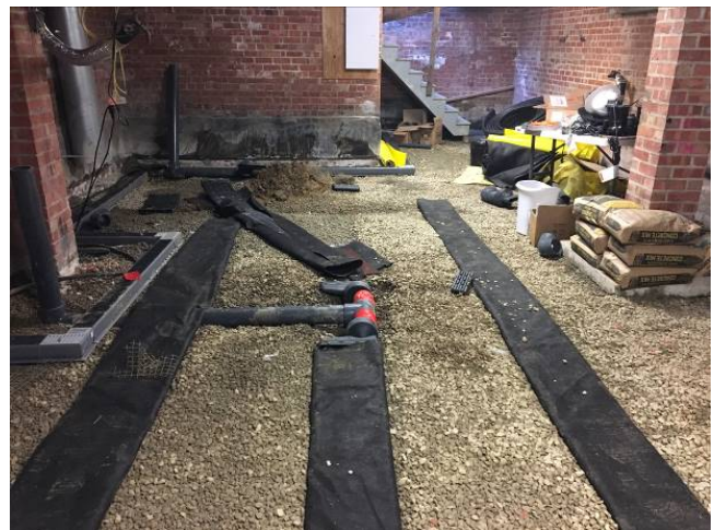
Photo 6: VMS Piping Installation
