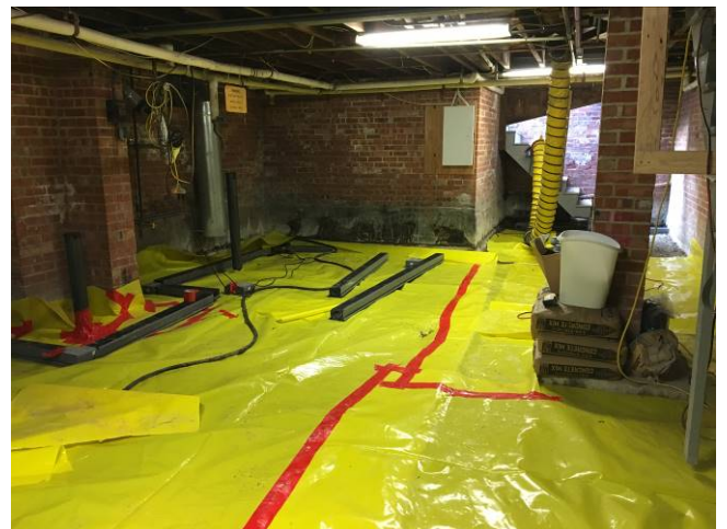
Photo 12: Vapor Barrier Installation
