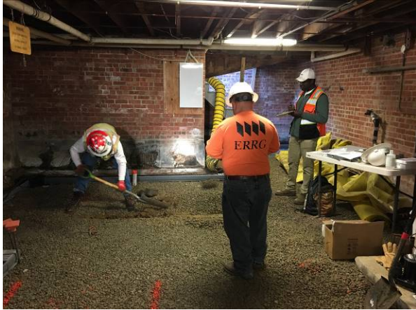
Photo 1: Initial VMS Layout and Trenching
