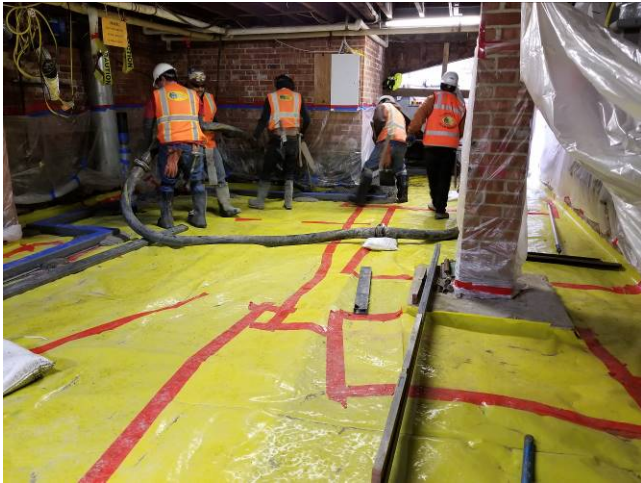
Photo 15: Concrete slab installation.
