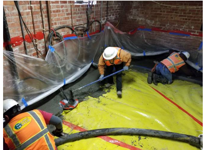
Photo 16: Concrete slab installation.
