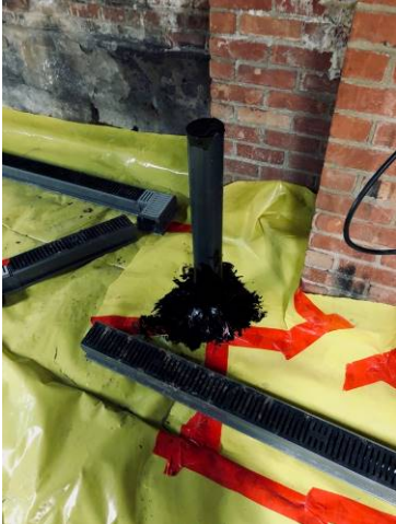
Photo 13: Vent Riser Penetration Sealing
