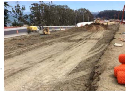
1325: Chavo continues pushing hort soil to the east. Hort is SP-56 and SP-57. Soil is consistent with horticultural soil from the stockpiles.
