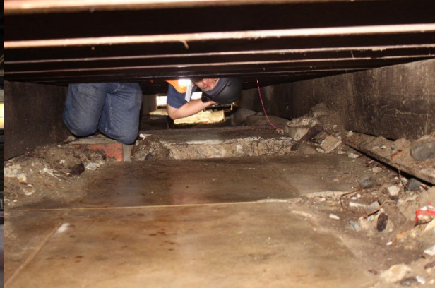
FIGURE 16: TRUST ARCHAEOLOGIST EDWARD DEHARO WITH 20TH CENTURY FEATURE IN CRAWLSPACE OF BUILDING 1185
