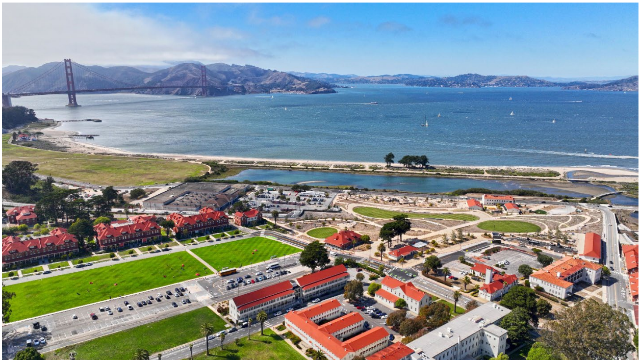
FIGURE 6: TUNNEL TOPS AERIAL, JULY 2022 (CHRIS CORNER, PRESIDIO TRUST)
