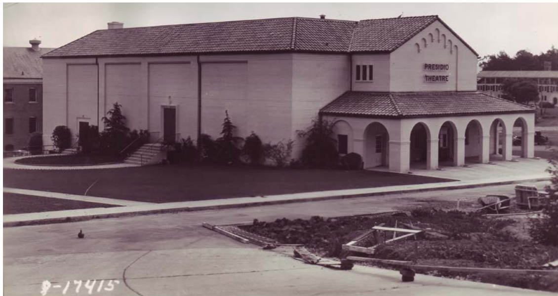
1.42 Presidio Theatre construction photograph of the completed east and south (main) elevations. Photograph clearly shows the upper story windows and mullions, the upper cornice concrete detail, and the metal lettering sign at the front of the building. (1939, NARA)
