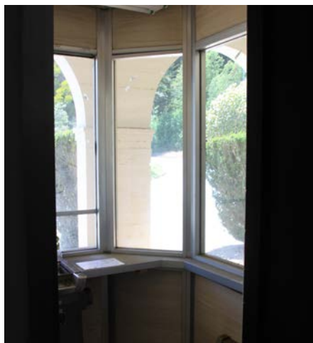
3.40 Aluminum frame Plexiglas windows replaced the original ticket booth windows in 1987. (2014, PT)
