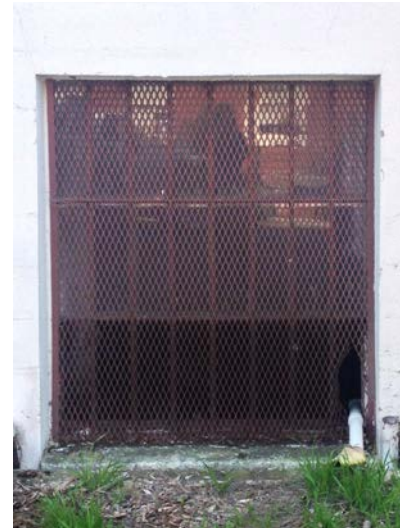
3.28 North elevation, basement window with metal grate. A hole made for utility piping attracts wildlife into the basement. (2014, PT)
