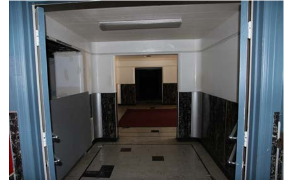
2.51 Room 06. West Foyer looking east from Entrance Hall showing blocked entrance to the private lounge on the left. Note the hardboard wainscot with aluminum curve detail. (2014, PT)
