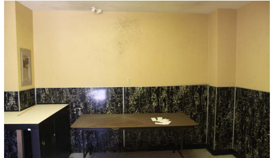
3.37 Mold and peeling paint on the north wall and ceiling in the west office suggests water infiltration. (2014, PT)
