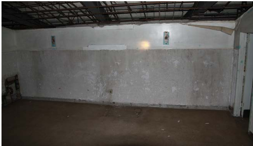
3.38 A composite tile flooring in poor condition remains in both lounges. It appears that all base boards were removed with much of the wall finish. (2014, PT)
