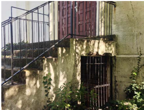
3.22 South auditorium stair on the west elevation is in very poor condition. The shaded and damp conditions have caused concrete failure. (2014, PT)
