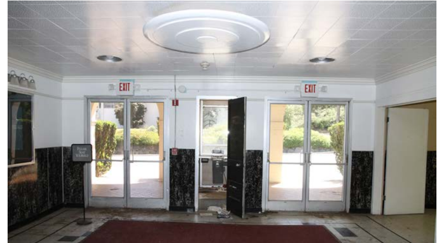
3.46 The lobby originally featured a plaster ceiling but is now covered in acoustic tiles; it is likely that the original ceiling is intact and can be restored. (2014, PT)
