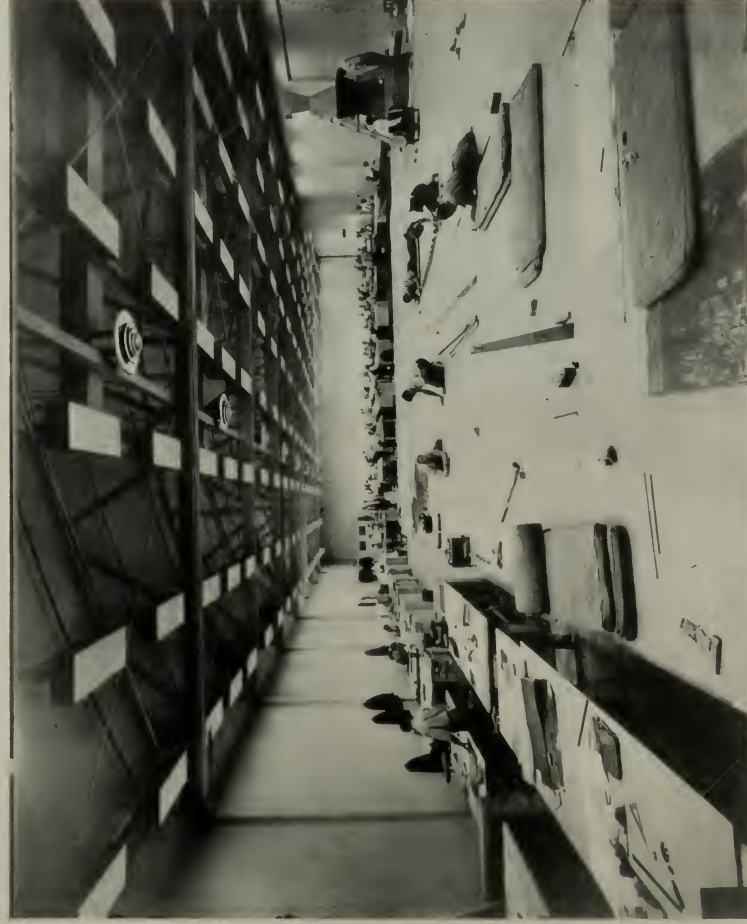
Air is distributed uniformly and without drafts over the vast floor area of this loft of the Vega Aircraft plant, at Burbank, California. By scientific air-diffusion, Anemostats (on the under-side of the trusses) insure equalization of both temperature and humidity.
