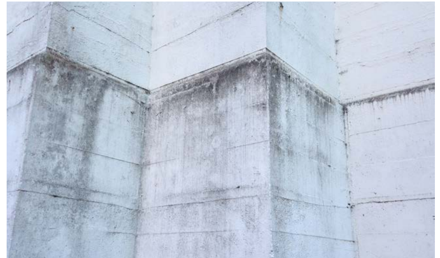
3.6 A detail of biological growth and soiling on north elevation. (2014, PT)
