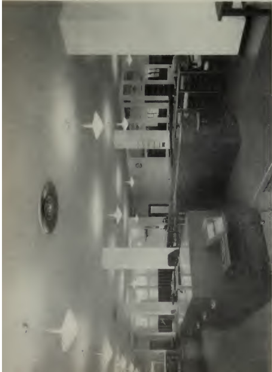
Air-diffusers insure uniform distribution of air throughout virtually all types of public buildings. Here in the Stanislaus County (California) Court House, these devices are seen on the ceiling.
