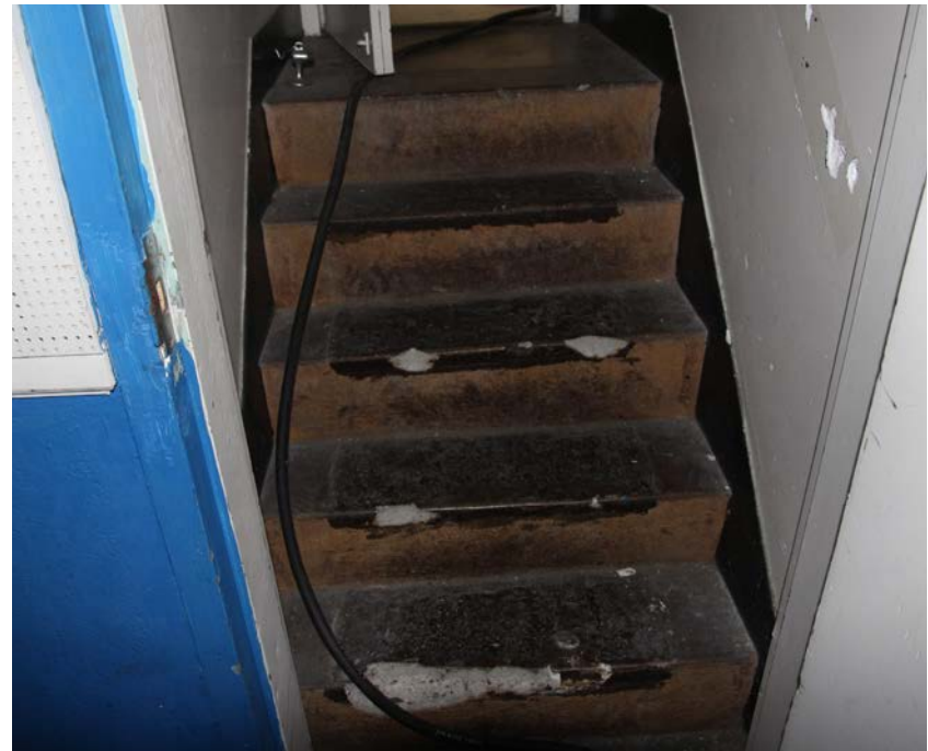
3.80 The concrete projection room stairs show loss of material and continued deterioration. (2014, PT)
