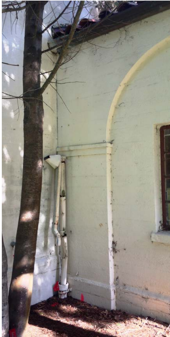
3.13 At this corner near the west office shows a dismantled downspout. (2014, PT)
