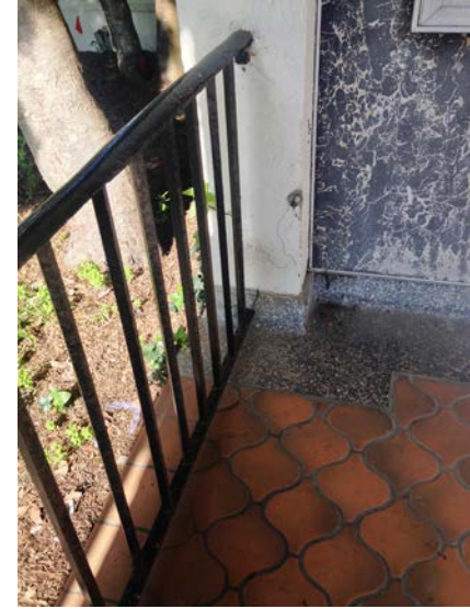
3.3 The northwest corner of loggia wall exhibits cracking and spalling at the connection point with the iron railing. (2014, PT)
