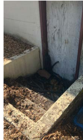
3.19 Debris in the east elevation, crawl space stairs. Plywood is covering the crawlspace opening. (2014, PT)
