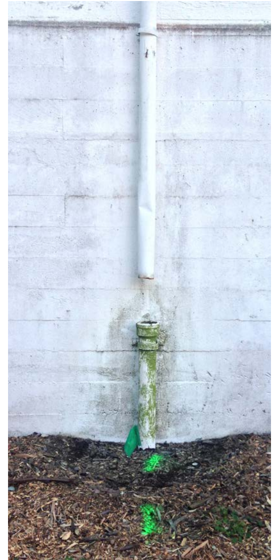
3.14 A portion of this north elevation downspout is missing. (2014, PT)
