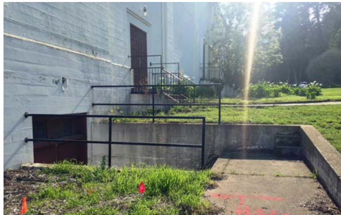
3.17 Basement iron tube railing is in good condition. The auditorium stairs on the west elevation can be seen in the background. (2014, PT)
