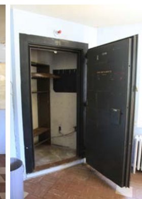
2.45 Room 05. Fireproof film vault intact and unchanged. (2014, PT)
