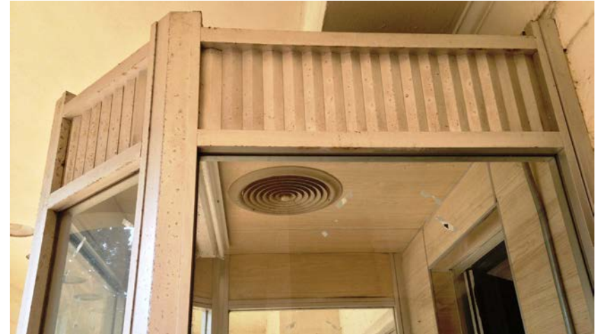
3.9 Ticket Booth Exterior is aluminum in fair condition. Although largely protected from the elements, the aluminum exhibits some pitting. (2014, PT)
