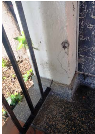
3.16 The railing and concrete connection shows signs of rusting and failure at the west end of the loggia. (2014, PT)
