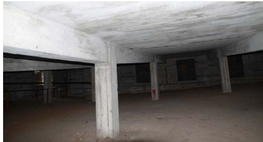
3.8 Interior of the crawlspace showing a dirt floor, concrete piers, beams and concrete foundation walls (background). (2014, PT)
