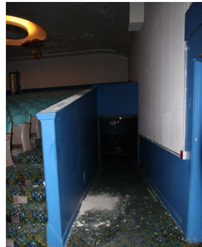
2.46 Room 10. West Entrance Hall looking south from auditorium showing acoustic tile on the perimeter wall (right). (2014, PT)
