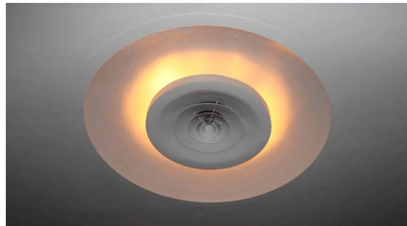
2.61 Room 12. Detail of one of six original light fixture and air handling unit. (2014, PT)
