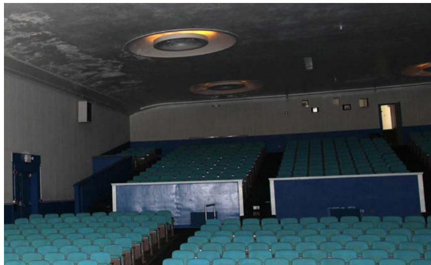
3.60 The partial height plaster-concrete partitions with a wood cap that separate the upper and lower seating sections are in good condition. (2014, PT)
