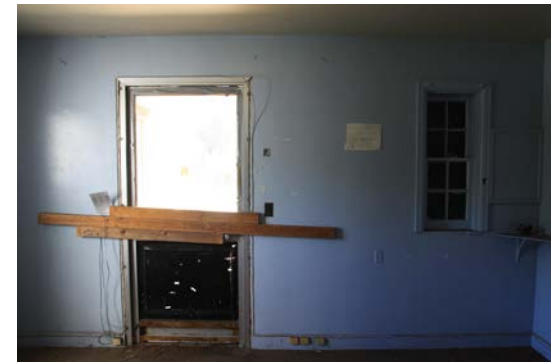
2.43 Room 09. (right) Office, south wall, showing 1962 storefront door with barricade. An original wood-frame window is intact but blocked by a poster case on the exterior wall. (2014, PT)
