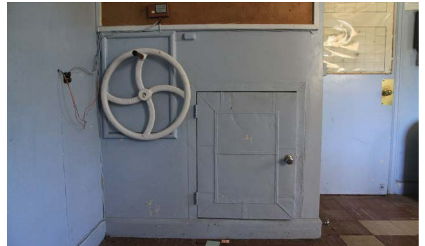
3.53 The wood-frame dumbwaiter with a metal shaft, metal door and elevator wheel is in fair to good condition. There is evidence that updates to the dumbwaiter included electrifying the system; it is uncertain whether the manual or electric systems are functional. (2014, PT)
