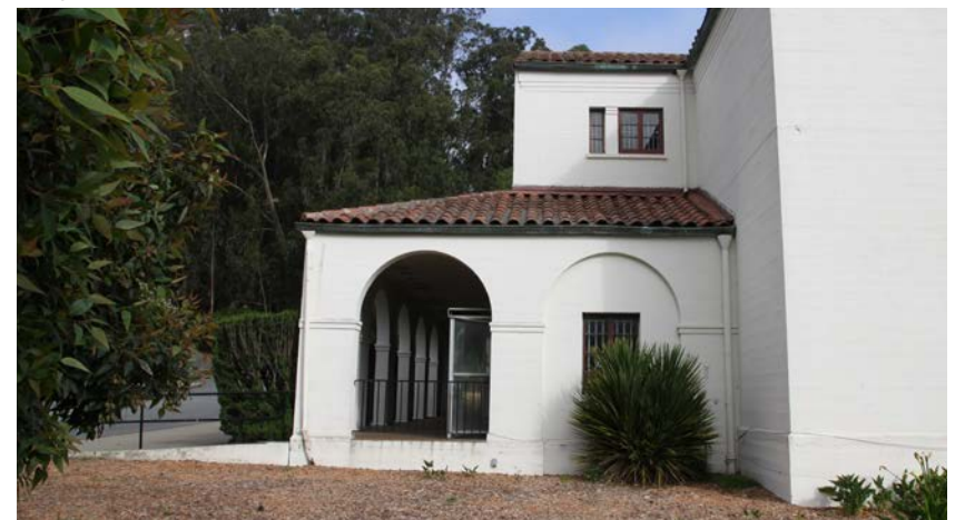
2.8 East elevation of the pavilion. Note the upper story windows where one mullion was removed and two windows were combined. (2014, PT)
