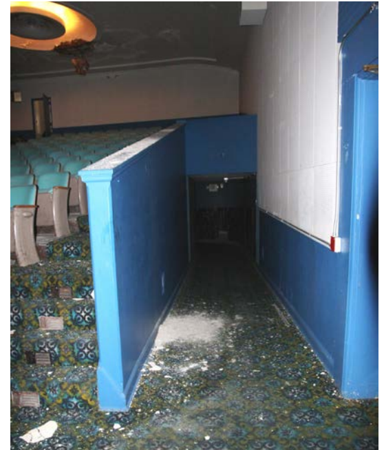
3.58 The stairs up to the upper seating area, looking south towards the west entrance hall. The plaster-concrete partial wall (left) and concrete wainscot (right) are in good condition. Fallen plaster from the ceiling has left small piles of white debris on the carpet. (2014, PT)
