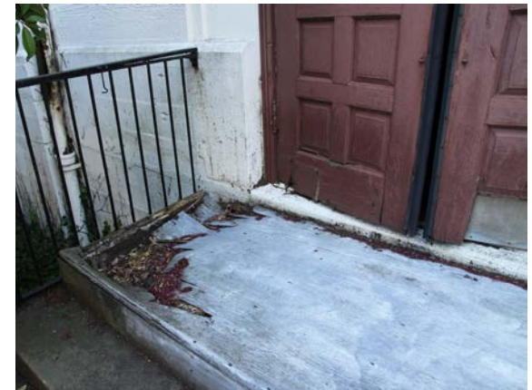
3.24 A failing plywood step added at the landing of the north auditorium stair on the east elevation. (2014, PT)
