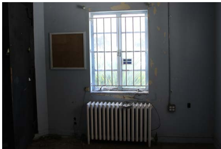
3.41 East office, double casement metal frame window with security bars attached to the inner sill. Deferred maintenance is evident around the frame and sill however all window panes are intact. (2014, PT)
