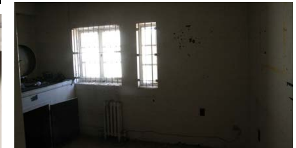
2.87 Room 15. Rewinding room window (east elevation). Note that only one mullion remains. There is no record of this change. (2014, PT)
