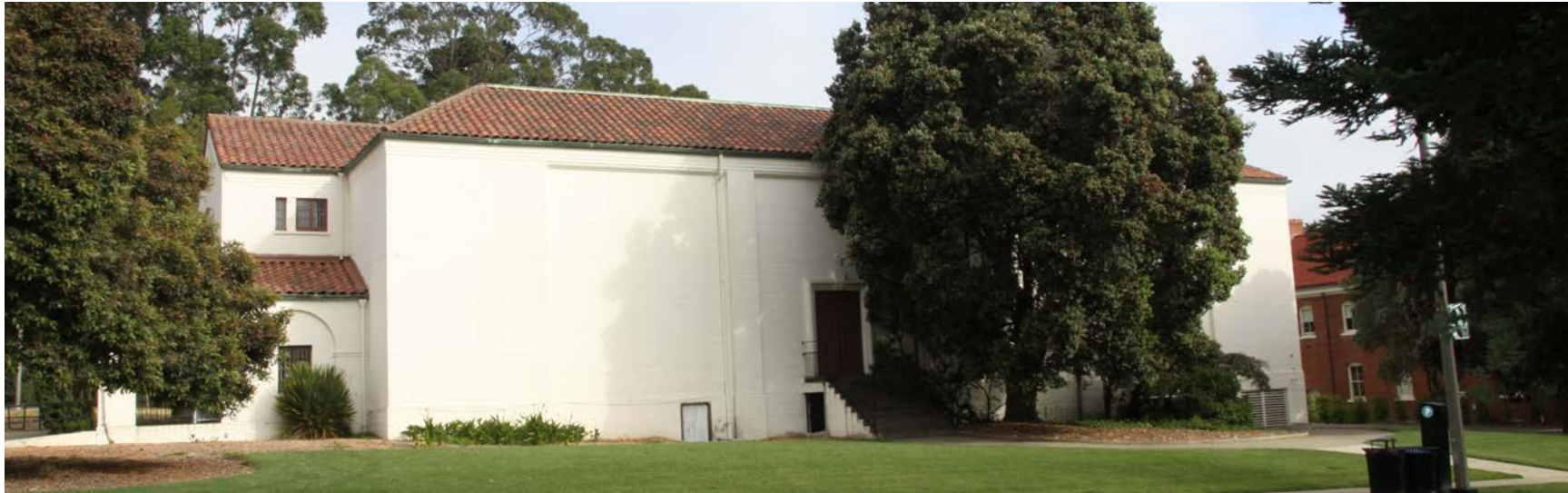
3.11 East elevation roof showing both the gable roof of the south elevation and the hip roof atop of the auditorium. (2014, PT)
