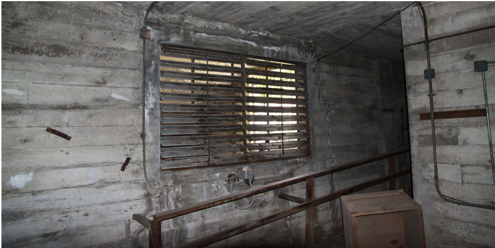
3.86 A vent showing signs of rust and deterioration is located at the east wall of the basement. (2014, PT)
