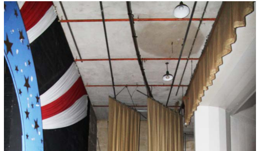
3.68 Water stains are visible on the stage ceiling. (2014, PT)
