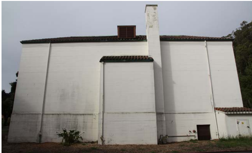
3.5 The dark coloring on the north elevation shown here is evidence of both dirt and biological growth on the exterior wall. (2014, PT)
