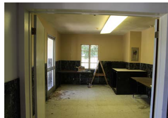
2.38 Room 04. Office looking west through the open double doors from the lobby. Note on the left, the 1962 aluminum-frame storefront door from the loggia. The original casement window is extant. (2014, PT)
