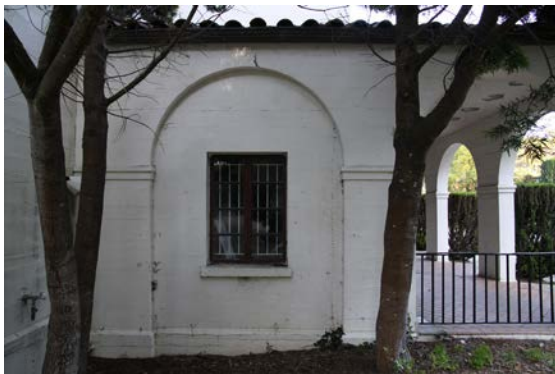
3.25 The west office has a metal frame double casement window with security bars installed on the interior sill. The same condition occurs on the east end wall of the east office. (2014, PT)
