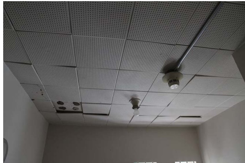
3.76 The missing or falling ceiling tiles in the western (generator) room is a typical condition found in each of the projection rooms. (2014, PT)
