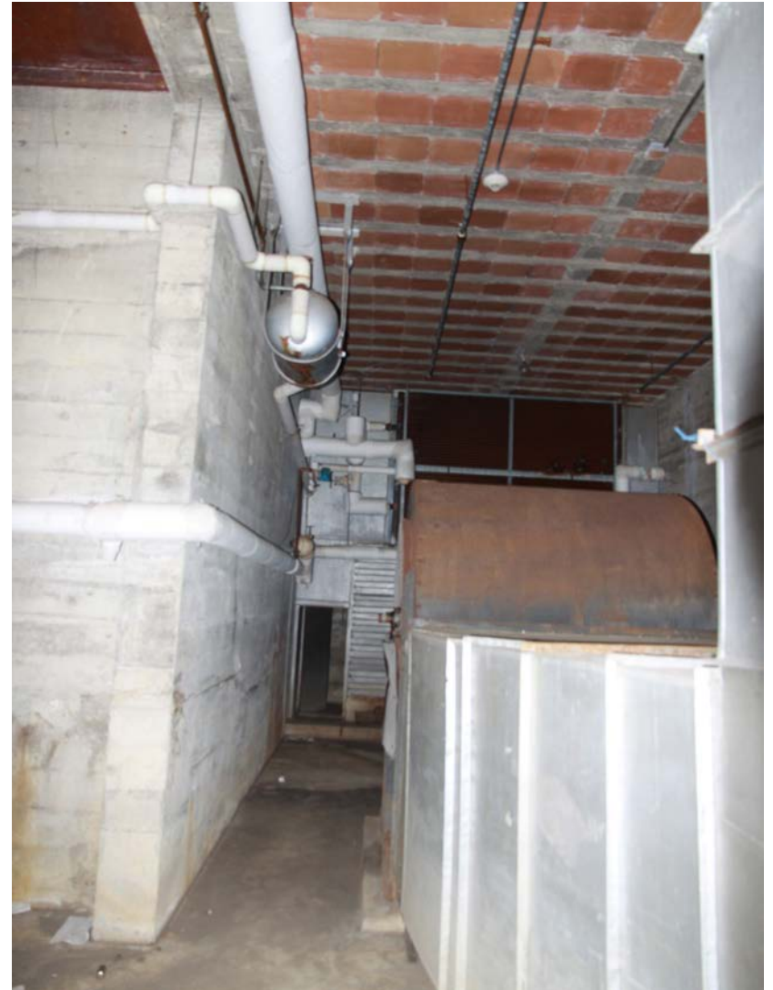
3.87 The exposed clay tile ceiling, unpainted concrete walls and unfinished concrete floors in the basement appear to be in fair condition. (2014, PT)
