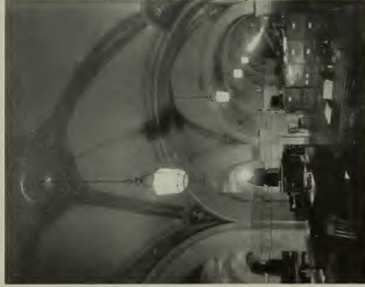
Only scientific air-diffusion could afford proper air-distribution in this room with a vaulted ceiling. Here at the Bank of America, Los Angeles, air enters the room through Anemostats. Lighting fixtures are suspended from each of these air-diffusers.
