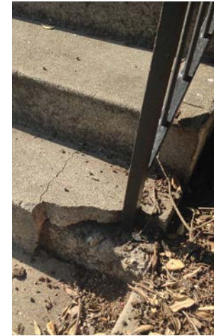
3.20 Failing and missing concrete at the bottom of the south stairs on the east elevation. (2014, PT)
