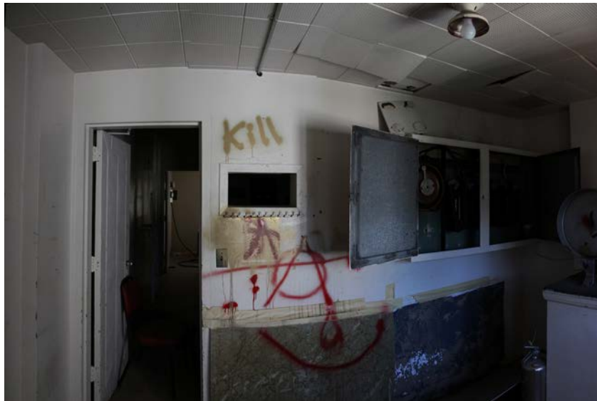
3.75 The eastern projection room contains a mix of finishes and some graffiti. The west wall of this room features original plaster walls with hardboard wainscoting haphazardly attached (or detached) from the wall. (2014, PT)
