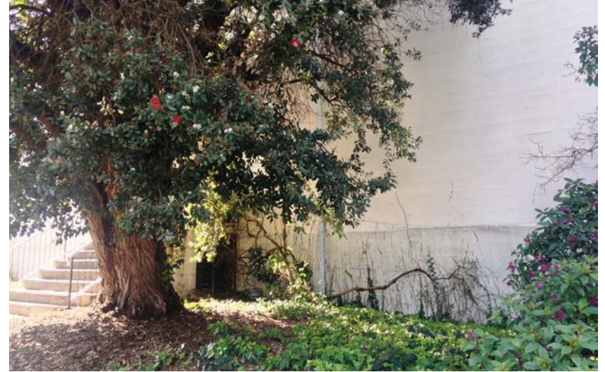
3.4 Current and past evidence of damage caused by foundation plantings can be seen on the east elevation. (2014, PT)
