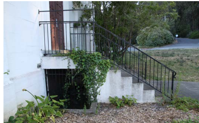
3.18 At the west elevation auditorium stairs, an iron railing was added to the top tube of the original railing, perhaps to stabilize the original railing. Security bars, partially obscured by vegetation, block the open space under the stairs. (2014, PT)
