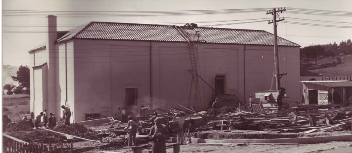
1.38 Presidio Theatre construction photograph of the north and east elevations near completion. Image shows laborers at work, the two auditorium exits with open doors, and a nearly completed roof. (c. 1939, NARA)
