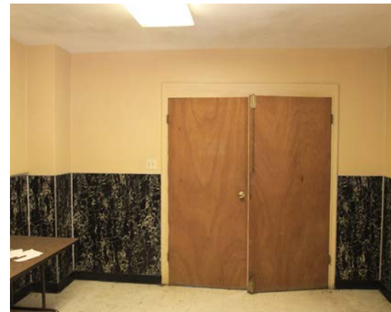
2.37 Room 04. Office interior looking east. The room retains the 1962 wainscot and rubber base. The single door was later widened to a double door after 1962. (2014, PT)
