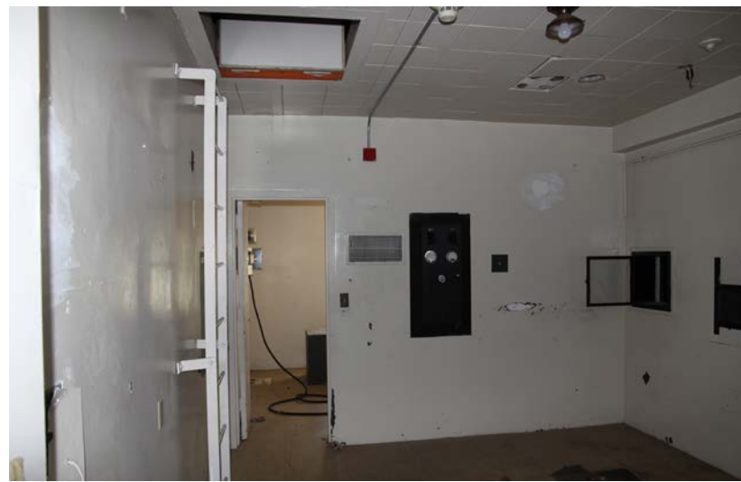
3.83 The original metal ladder (left) provides access to a hatch leading up to a catwalk. (2014, PT)
