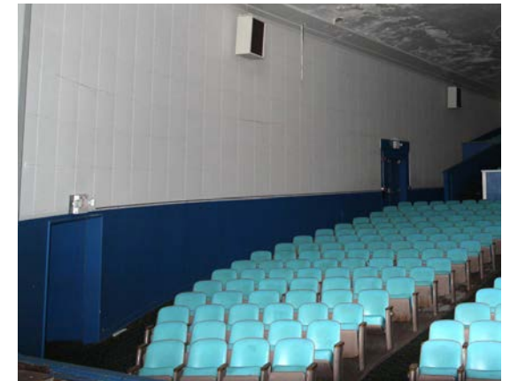
2.67 Room 12. East wall of the Auditorium showing the current acoustic tile finish above the original plaster finish. (2014, PT)
