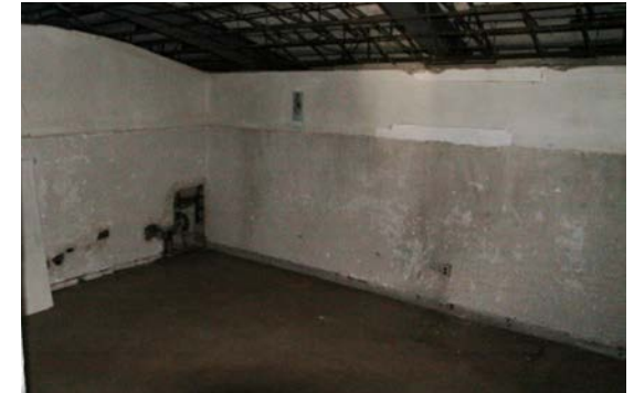
2.59 Room 09. Northwest corner of the east lounge showing that all wall and ceiling finishes were removed. (2014, PT)
