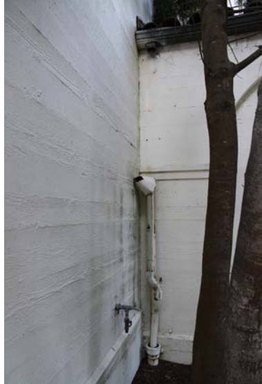
3.1 Board form finish exterior walls. (2014, PT)
