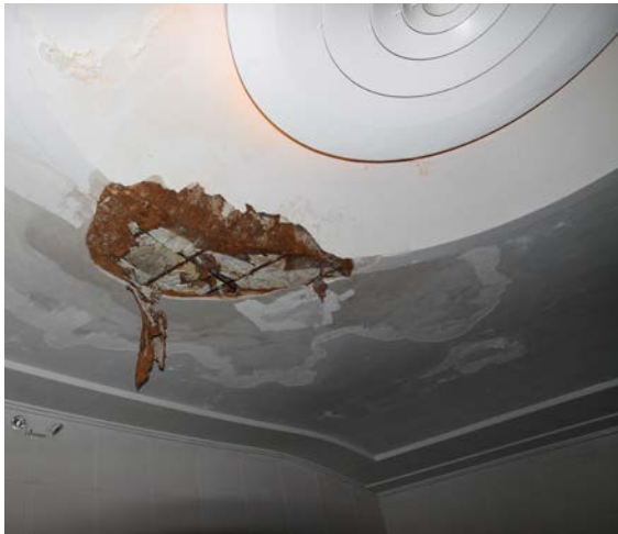
3.63 Missing plaster and lath at the southwest corner of the auditorium. (2014, PT)
