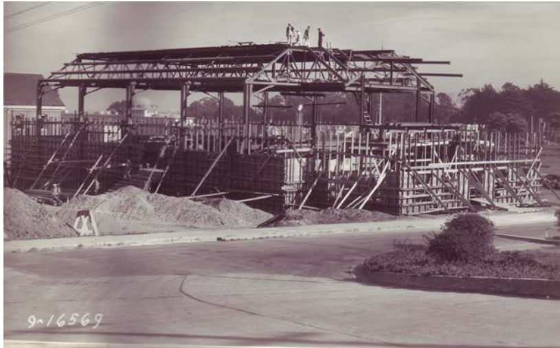
1.34 Presidio Theatre construction photograph documenting the erection of the auditorium steel truss frame, looking northeast. (c. 1938, NARA)
