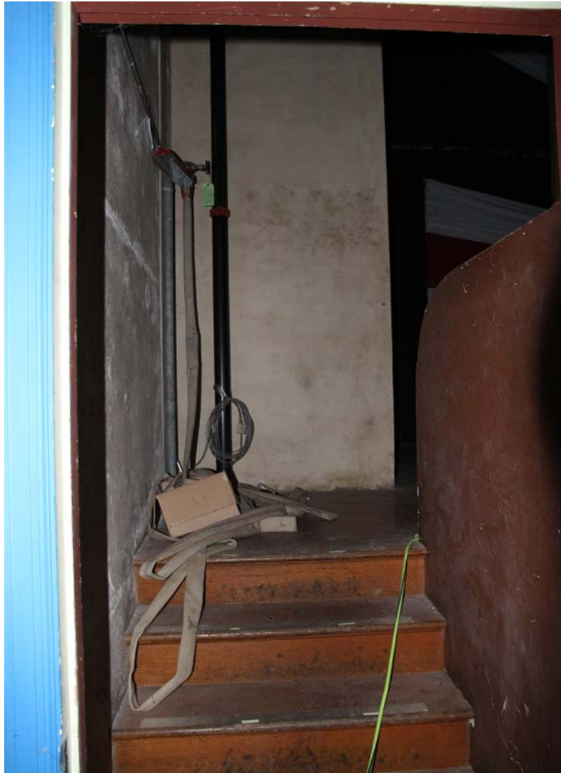
3.73 Wood stairs at the west end of the stage do not exhibit signs of dry rot and are in fair condition. (2014, PT)
