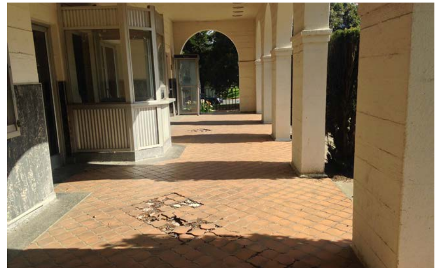
3.10 The loggia looking east. The delaminating and broken tile continues to worsen. (2014, PT)
