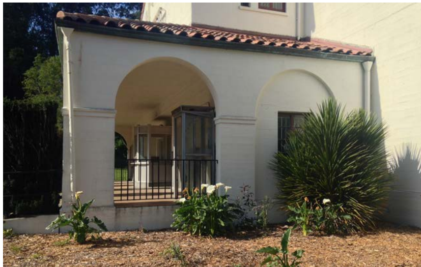
3.12 East elevation of the loggia shows an intact copper gutter and two functioning downspouts. (2014, PT)
