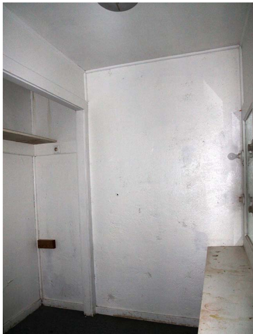
3.72 Dressing room contains vanities with lights, closets and lavatories. The walls are comprised of a post-war gypsum board with simple finishing. (2014, PT)
