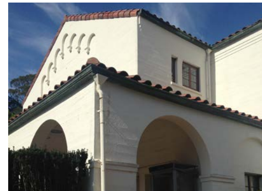
3.27 The upper windows on the east elevation are comprised of a single casement and a double casement metal frame windows separated by a single munnion. (2014, PT)
