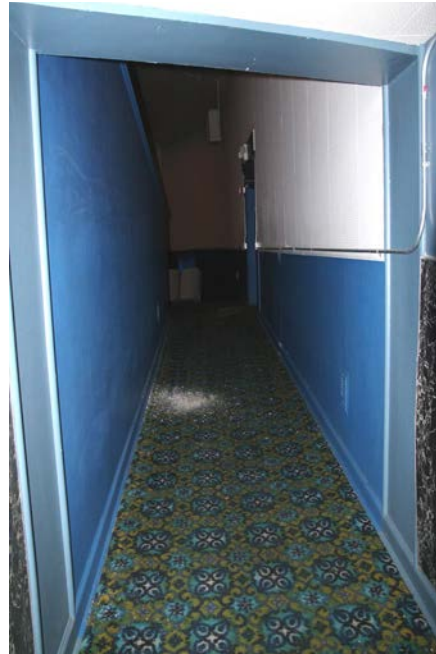
3.57 East entrance hall looking into the auditorium. On the other side of the partial height plaster-concrete wall (left) is the upper seating area. An acoustic tile wall over a concrete wainscot (right) that extends along the length of the wall. (2014, PT)
