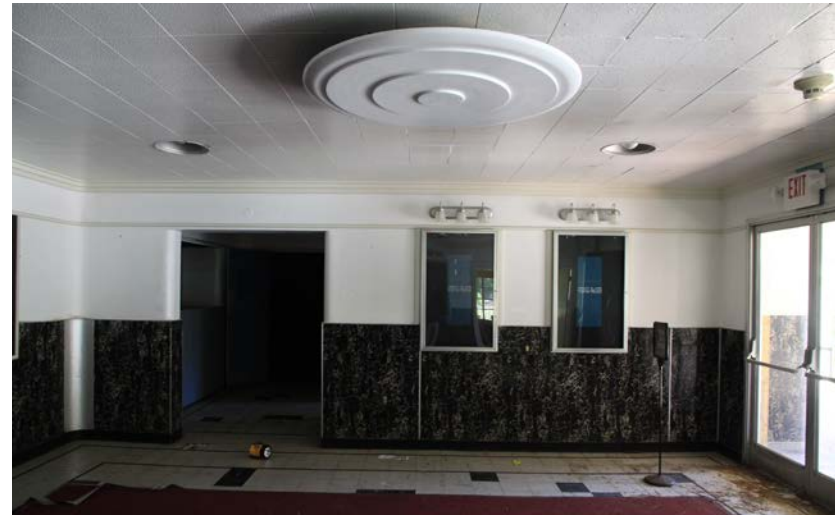
3.48 Flush single bulb lights in the lobby ceiling are likely original and should be kept. The Lobby also features several non-historic sconces over display cases that appear to be in good condition. (2014, PT)
