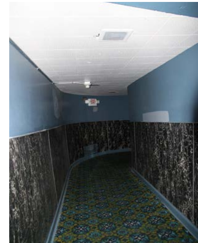
2.47 Room 10. West entrance hall looking west, curving south. Note the acoustic wainscot and the acoustic tile ceiling. (2014, PT)
