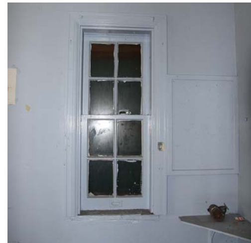
3.42 The east office wood frame window is in good condition but currently blocked by a poster case attached to the exterior wall of the loggia. (2014, PT)
