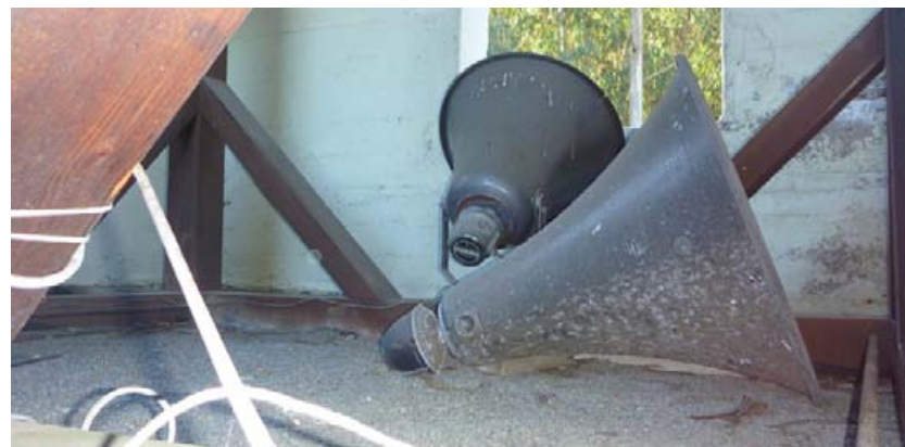
Horn-style loudspeakers in bell room; note condition of roofing and deteriorated wall surface.
