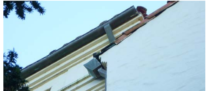
Typical gutter and downspout assembly.
