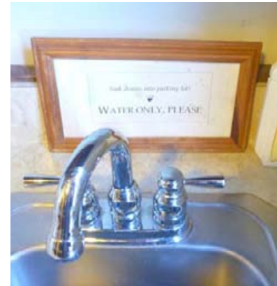
Vestry sink; note sign that says "Sink drains into parking lot! Water only, please"
