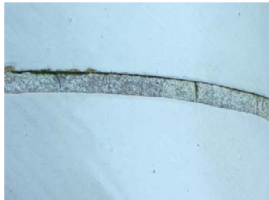
Example of terra cotta mortar joint
