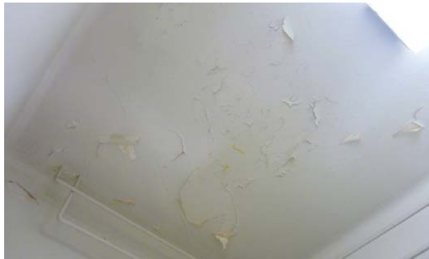
Delaminated paint on kitchen ceiling.
