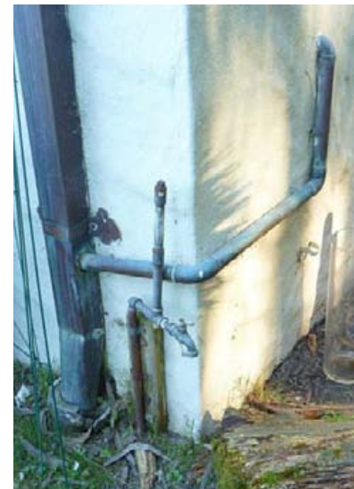
Vestry sink draining into copper downspout.
