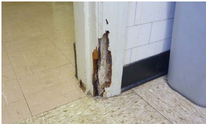
Rotted restroom door frame; also note asbestos floor tile.
