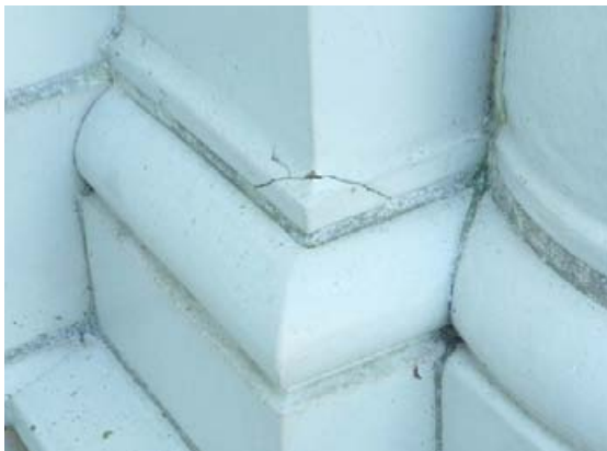
Cracking at base of terra cotta column.
