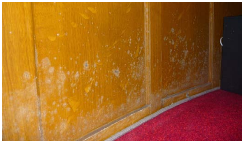
Mold and delamination on wood wainscoting in the chancel.
