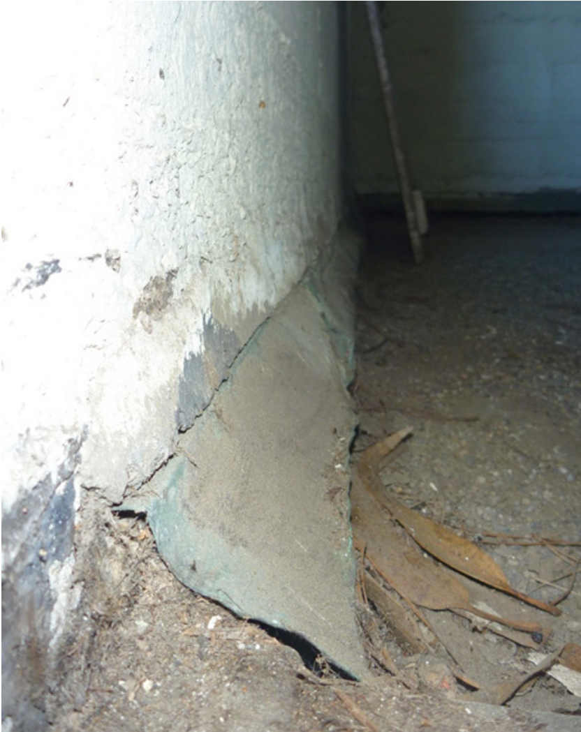
Deteriorated condition of roof flashing in bell room at the top of the bell tower.
