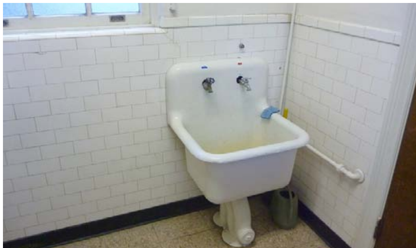
View of lower level restroom; note historic sink, cracked historic porcelain tile wainscoting, and double-hung window.
