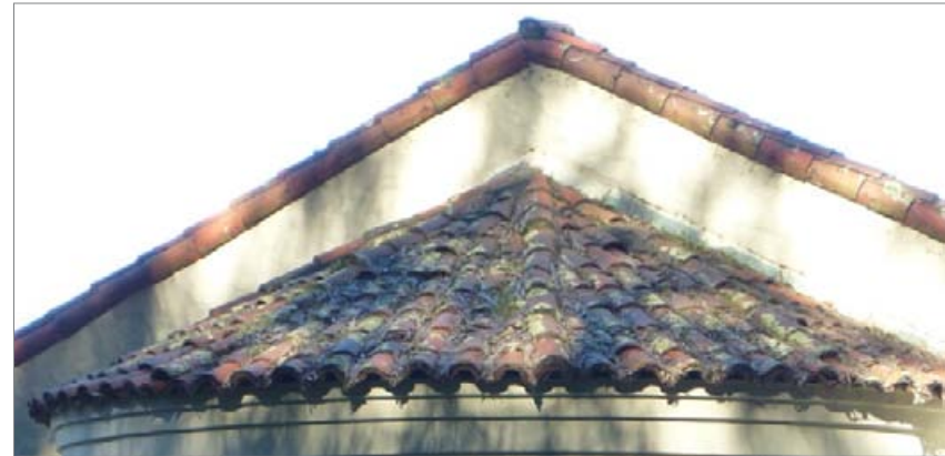
Condition of chancel roof; note absence of gutters and downspouts.
