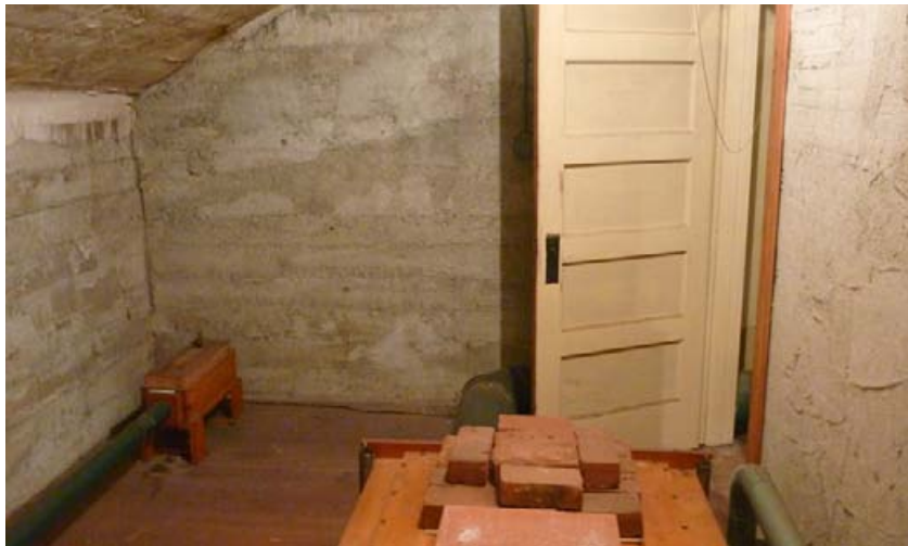
Ancillary room off the organ pipe chamber; note unfinished concrete walls and ceiling, as well as the five-panel wood door.
