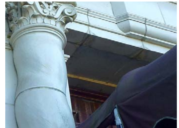
Detail of main entry door; note white stains due to water telegraphing down through terra cotta joints above.
