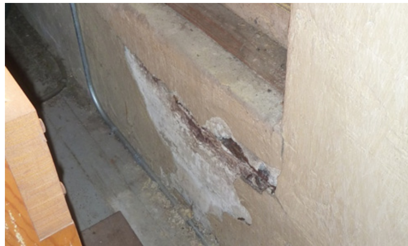
Organ pipe chamber window with spalled plaster and corrosion below.
