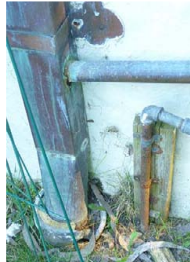
Downspout boot entering cracked drop inlet; note corrosion at downspout and plumbing union.
