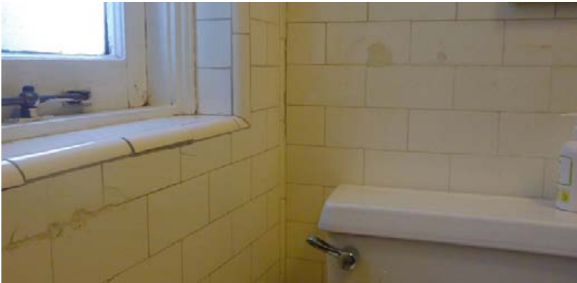
Patched and broken porcelain tile wainscoting in upper level restroom.
