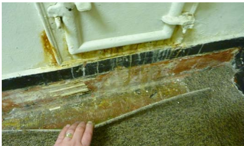
Efflorescence and staining from ashpit door.
