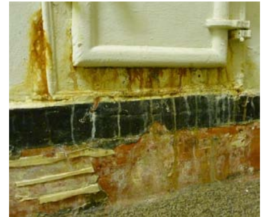
Efflorescence and staining at ashpit door.
