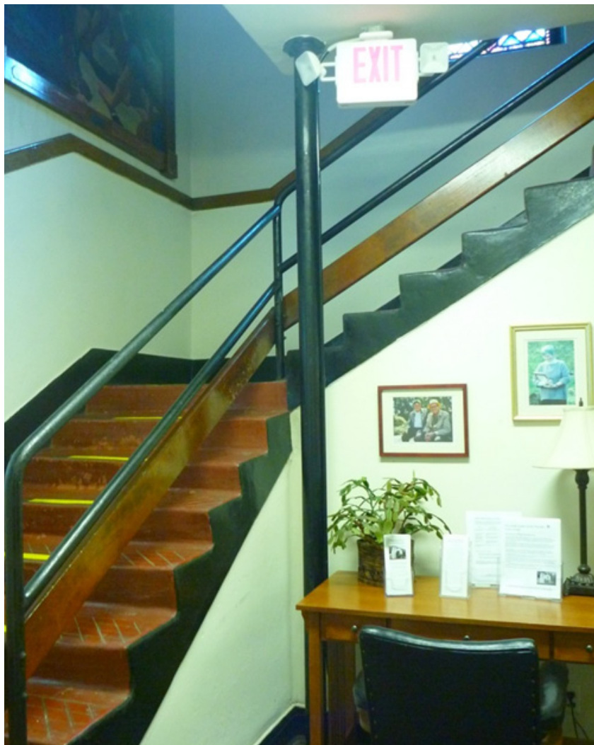
Lower bell tower stairwell; note height of handrail, 3" support post, and exit sign.
