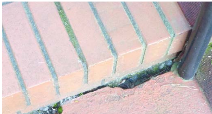
Mortar gaps at base of the main entry stairs.
