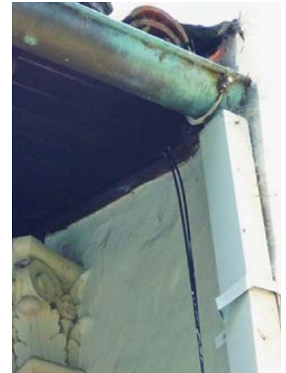
Example of inadequate intersection of gutter and downspout.
