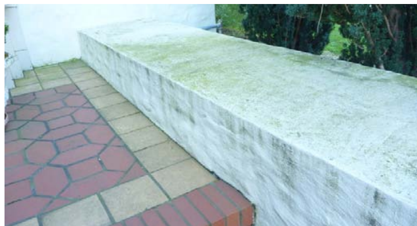
Example of biological growth and staining on stucco retaining walls flanking the main entry.
