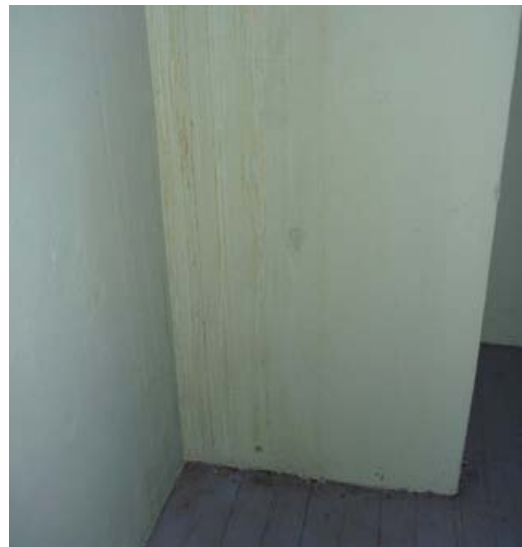
Water staining along chimney mass in bell tower.
