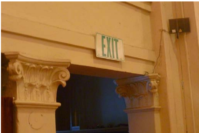
Example of unilluminated exit sign and cast stone capitals.
