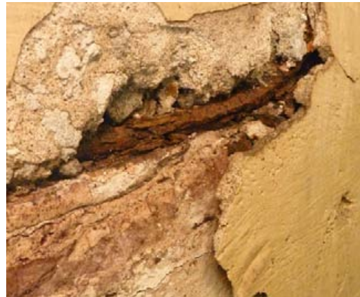
Example of corrosion and spalling in organ pipe chamber.
