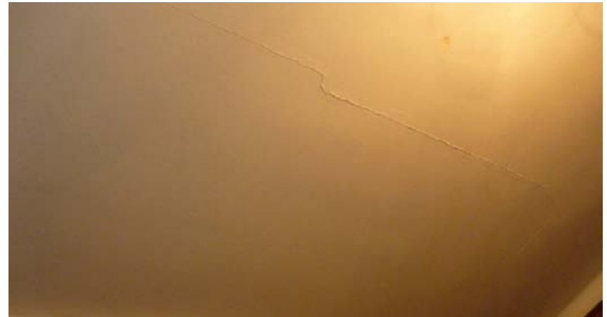
Ceiling crack in bride's room, caused because plaster has detached from the lath.
