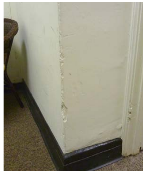
Impact damage to interior corners of boiler room hall.
