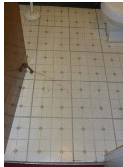
Note condition of worn vinyl flooring in upper level restroom.
