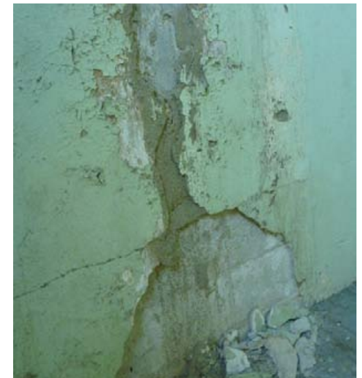
Efflorescence and spalling in bell tower.
