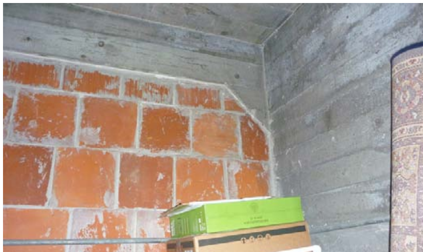
Boiler room walls: board form concrete and clay tile.
