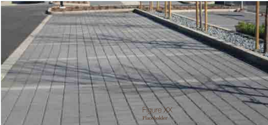
Figure 3-K Permeable paving and bioswales in parking lots allows filtration and minimize stormwater runoff.
