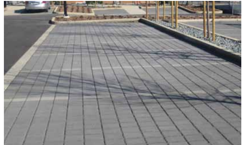
PERMEABLE SURFACES WILL ALLOW INFILTRATION AND MINIMIZE STORMWATER RUNOFF
