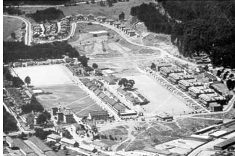
CONSTRUCTION FRAMING THE PARADE GROUNDS
