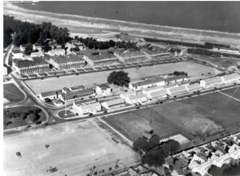
CONCEPTUAL DESIGNS FOR THE LODGE RECALL THE FOOTPRINT OF THE BARRACKS THAT ONCE LINED GRAHAM STREET. THE LODGE WILL RE-ESTABLISH THE DEFINITION BETWEEN THE TWO PARADE GROUNDS.
