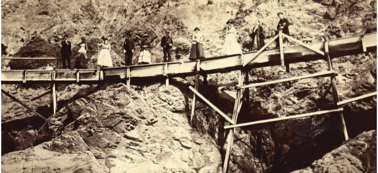
Circa 1870: A wooden flume walkway on the Presidio's Coastal Bluffs carried Lobos Creek water to the base of Van Ness Avenue to provide fresh water for the growing city of San Francisco.
