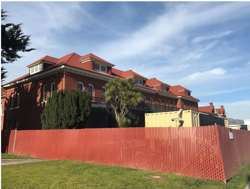
Building 105 showing off a new roof (M. Taylor)
