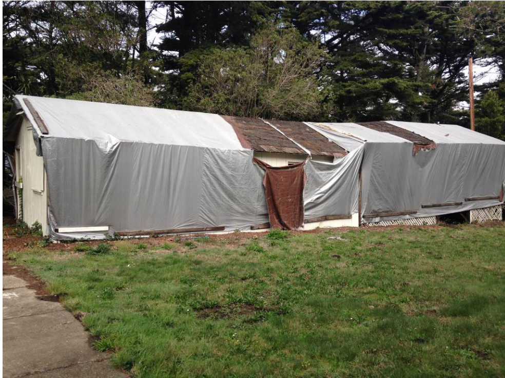
1390 prior to building stabilization work in 2017 (M. Taylor)
