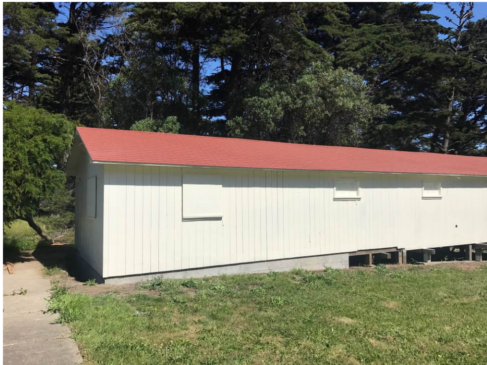
Building 1390 following completion of envelope repairs and structural stabilization (M. Taylor)
