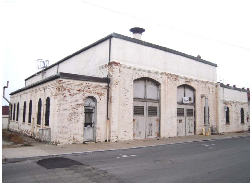
Building 1040, former powerhouse before deferred maintenance in 2015.
