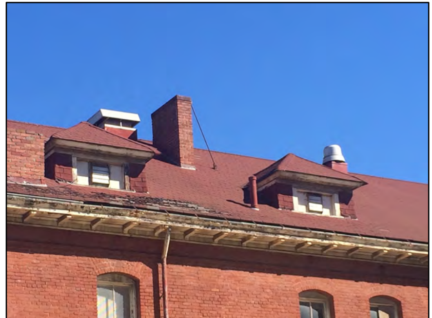
The brick chimneys have been reduced in height, capped, strapped and braced.
