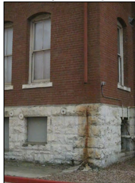
Below: Staining where downspout is missing
