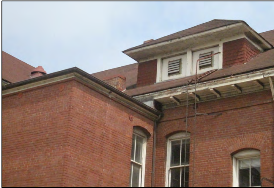
A detail of the intersection of the former stair tower with the main roof and rear dormer.
