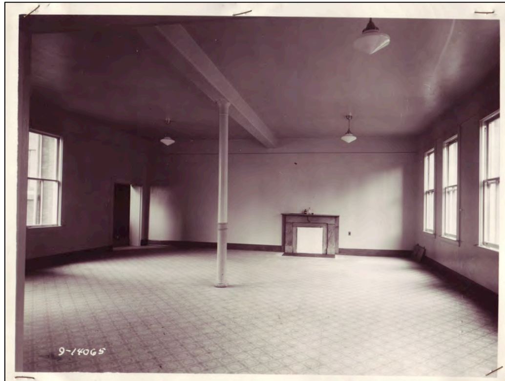
Interior view of Montgomery Barracks at the time of repairs, dated circa 1930s. Note materials, floor tile and marble surround at fireplace. Source: Presidio Trust Library.
