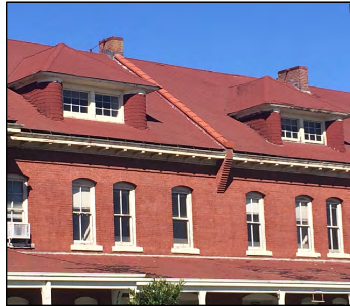
The dormer windows at the front elevation are in fairly good condition.
