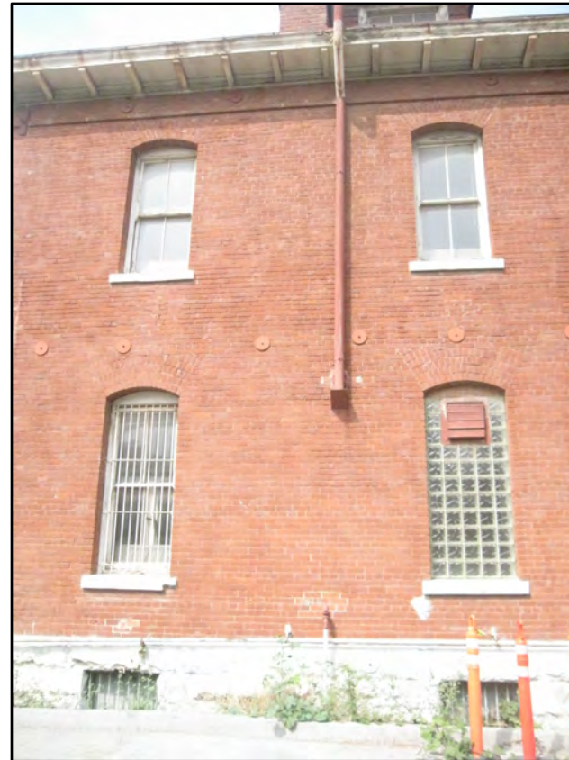
A detail of the south elevation showing one of the windows that has been infilled with glass block inserted at an unknown date.
