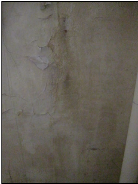
Plaster damage near stair 104
