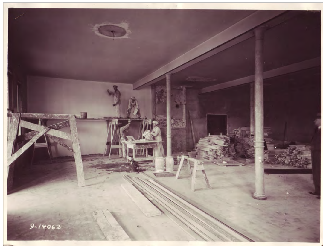
View of Montgomery Barracks, dated circa 1930s. Note plasters at work and original baseboards and trim to be reinstalled. Source: Presidio Trust Library.
