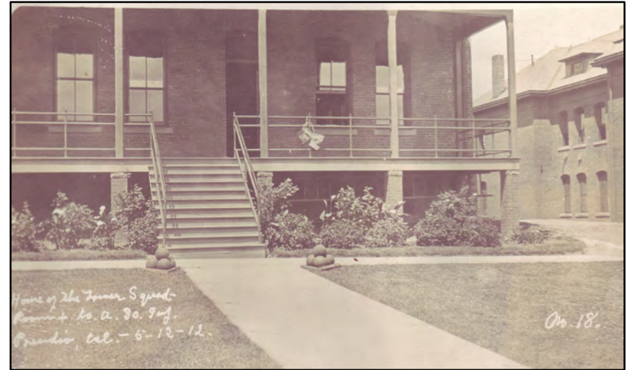
Above: A detail showing the corner of the east veranda of one of the Montgomery Street Barracks (not Building 105). However, the image shows how the porch posts and brick piers align and illustrates the early landscaping techniques to mask the area under the veranda. Source: Tucker Beckett Collection, PTL, May 12, 1912.
