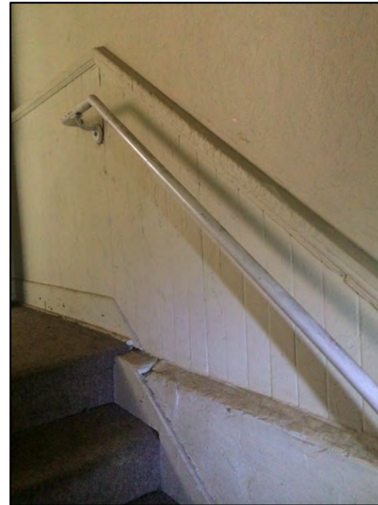
Above: The basement stair at the south side of the building retains some original wood wainscoting and a railing.
