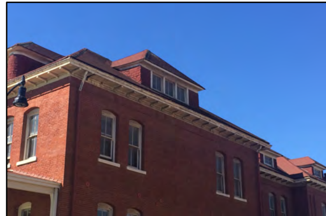
Below: The north façade dormer that replaced the north chimney. A north wing dormer is visible in the far right of the picture. These dormer are smaller than the dormers of the main roof.
