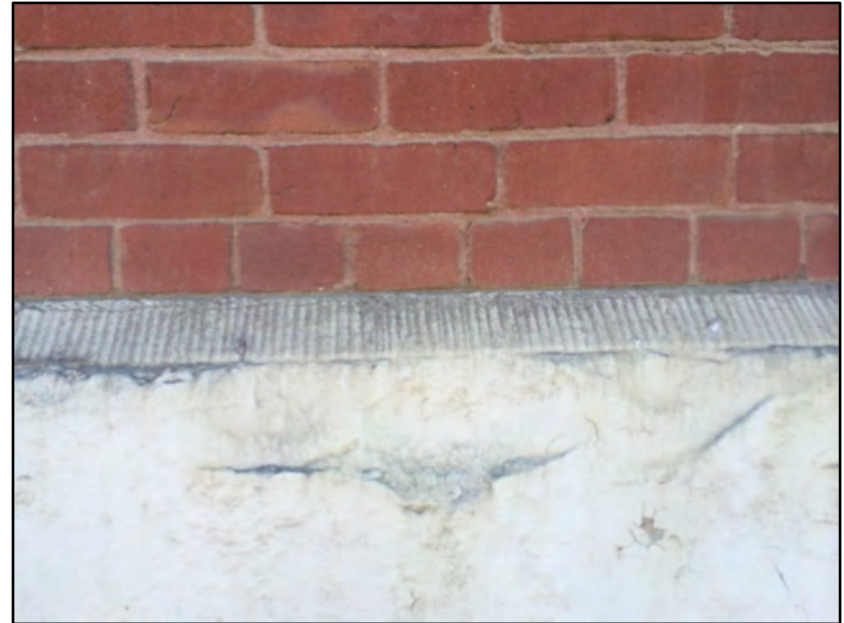
Above: A detail of the sandstone lip above the rough faced foundation veneer at the north elevation.
