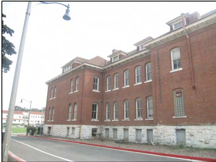
The punched openings of the basement windows along the north elevation. Note the boards covering the windows as a security protection measure. This occurs in all basement window locations.
