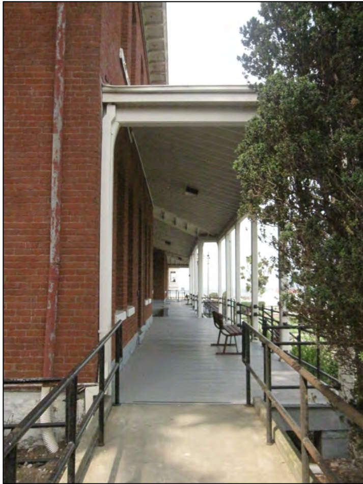
A detail of the front veranda stairs and railings. Note the replacement stair railings are heftier than the original railings which remain at the veranda.
