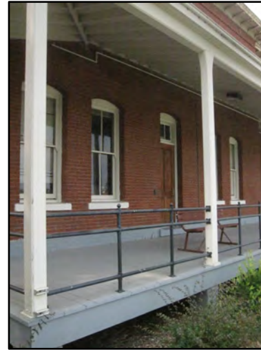
Above: Detail of the metal rail connection to the chamfered posts Below: The reconstructed stairs to the single entry at the south end.
