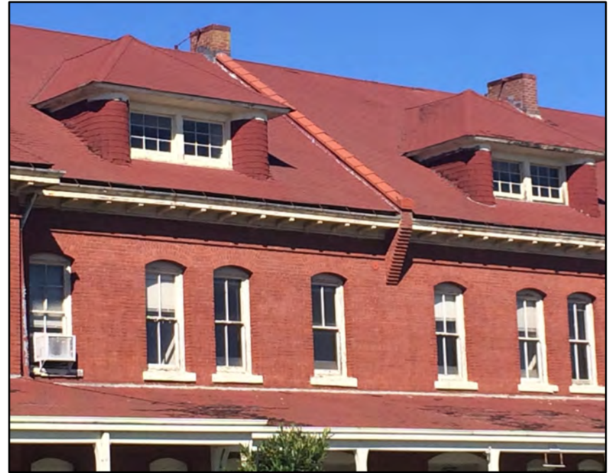
A detail of the east façade showing the corbeled and tiled cap to the brick dividing wall and the rounded edge of the dormers.
