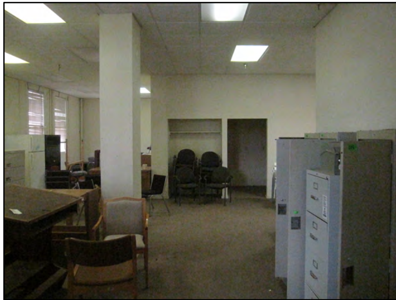
Above: Room 112 on the first floor showing the boxed in cast iron column. Left: A detail of the wood baseboard that remains mostly at the interior locations of perimeter walls.
