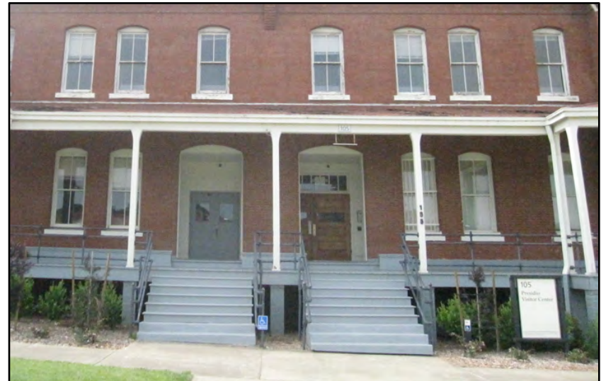
The twin front entries of all of the Montgomery Street Barracks were altered by the Army on several occasions. The exterior doors were removed leaving the secondary interior vestibule doors.
