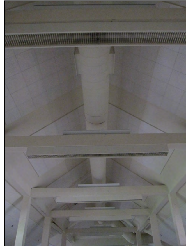
Above: The Queen's Truss system where it meets the apex of the roof.
