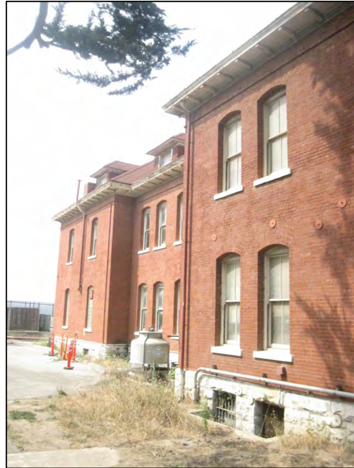
A current view of the south elevation, looking westward. Notice the window wells for the basement and the brick arches above the windows at the first and second floors, both character-defining features.
