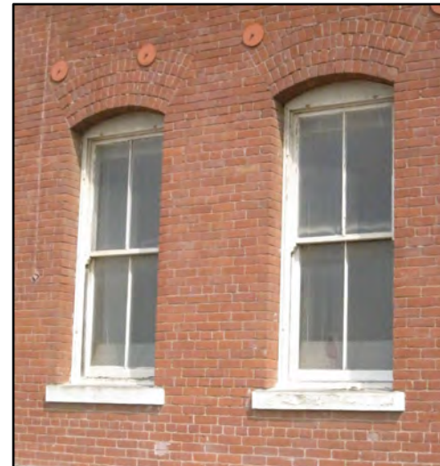
Typical exterior brick wall surfaces. Common bond pattern with arches above windows. Areas of repointing can be seen in some locations.
