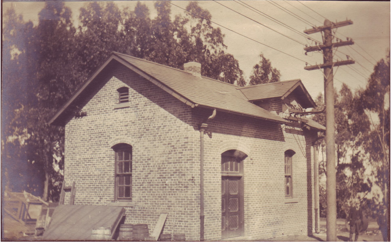
FIGURE 4: HISTORIC SUBSTATION BUILDING 107, SHOWN HERE IN 1913
