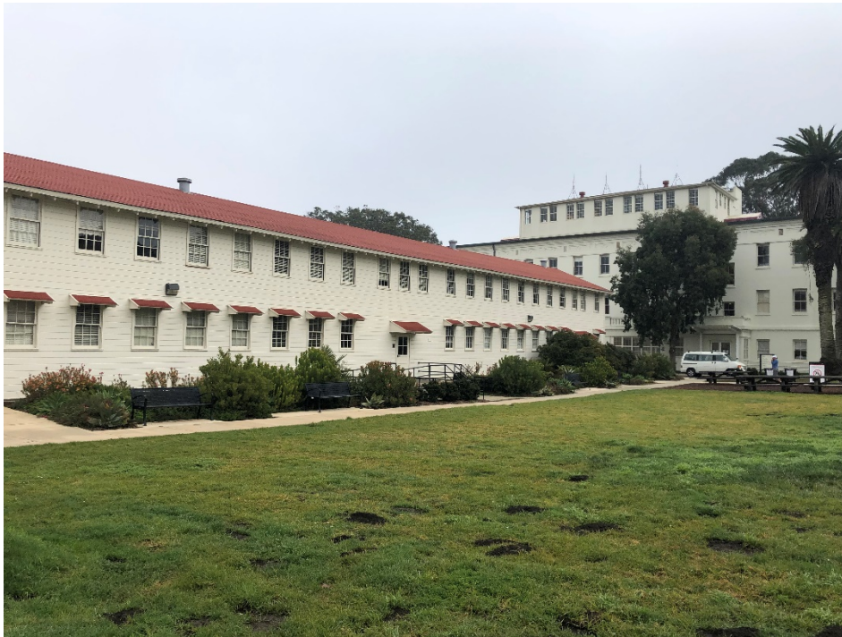
FIGURE 3 BUILDING 37 EXTERIOR REPAIRS
