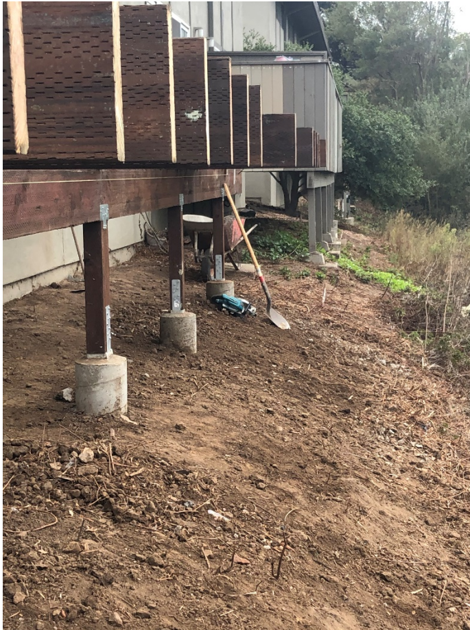
FIGURE 4 SANCHES DECK REPLACEMENT
