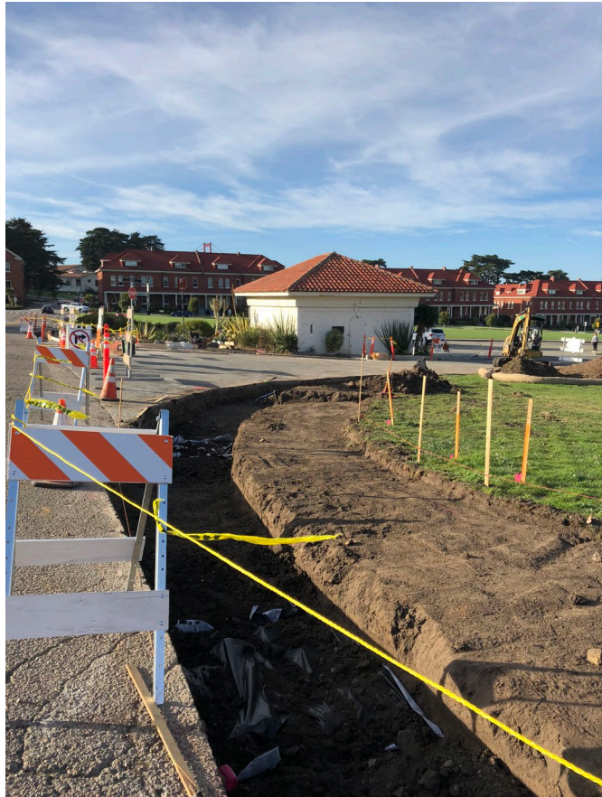
Figure 10 Sidewalk Construction along Graham (Presidio Trust, November 2018)
