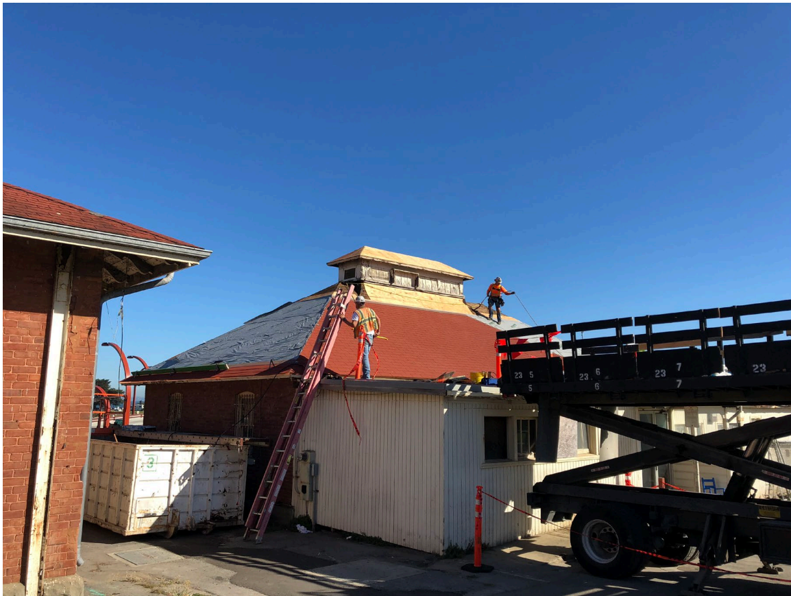
Figure 11 Reroofing Building 229 (Presidio Trust, November 2018)
