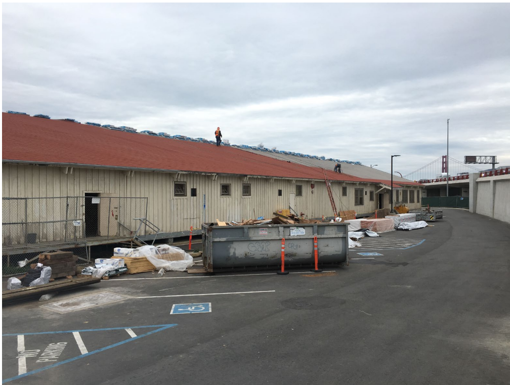
Figure 15 Building 1167 Rehabilitation (Presidio Trust, 2018)
