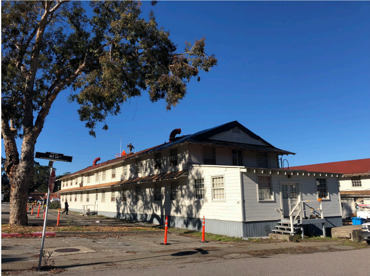
Figure 12 Reroofing Building 41 (Presidio Trust, December 2018)
