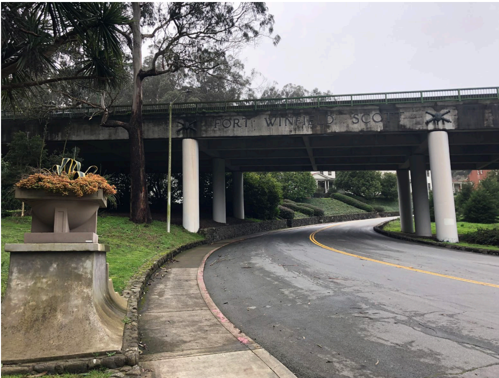
Figure 3 Fort Scott Entrance (Presidio Trust, January 2019)
