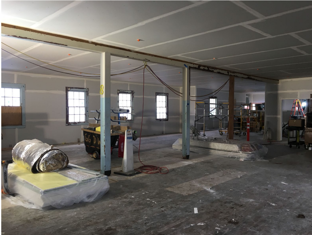
Figure 14 Building 1160 Rehabilitation (Presidio Trust, 2018)
