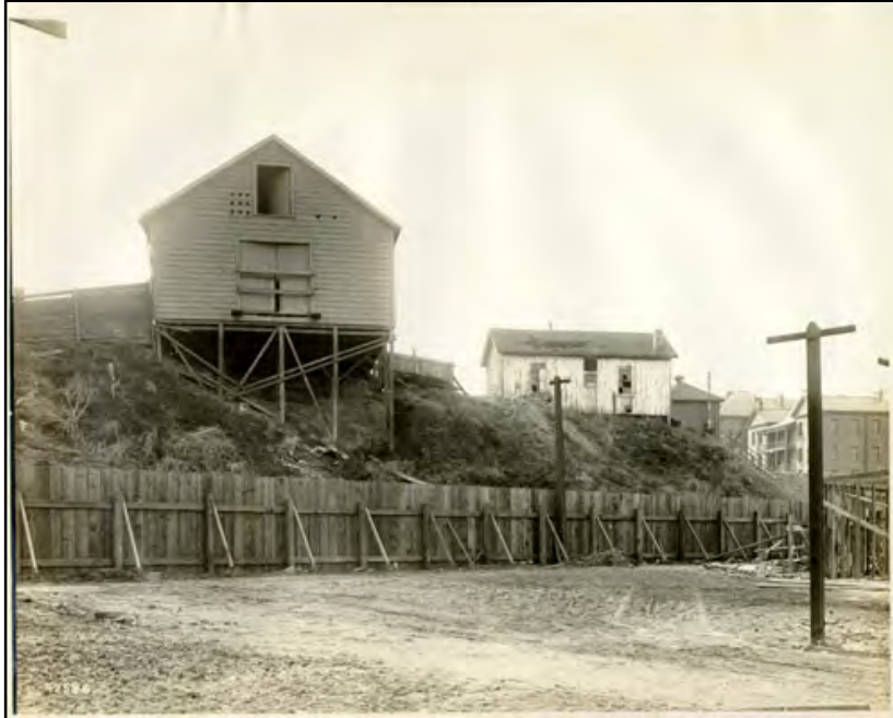
Figure 9. Quartermaster Complex, Cavalry Stable (Bldg. 44) on left shop on right, view southeast. Note post and pier construction. Photo courtesy of Presidio Trust
