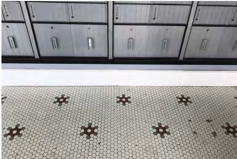
The newly exposed original tile floor in the current US Post Office at building 558. (M. Taylor)
