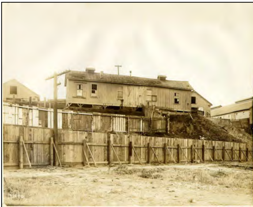
Figure 10. Quartermaster Complex, shop in foreground with Cavalry Stables (left Bldg. 46, right Bldg. 73) in rear, view southeast. Note post and pier construction. Photo courtesy of Presidio Trust.
